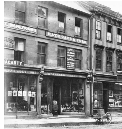
Figure 2: 1871 photo of Everett Bros. Hats, Caps and Furs, at their 100 Granville Street location.
