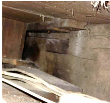
Figure 3: Photo showing the subject dwelling's timber frame construction with a mortise and tenon joint.
