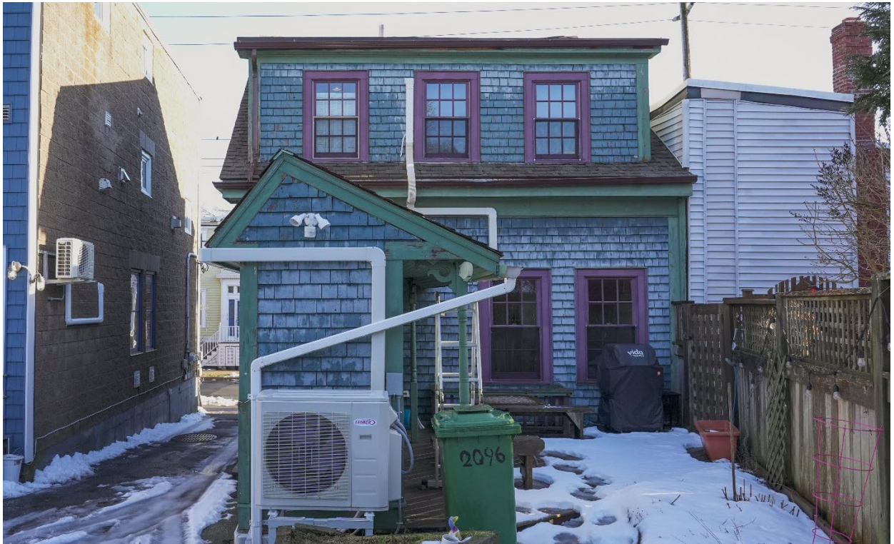
Figure 17: Western elevation (Feb. 15, 2023)
