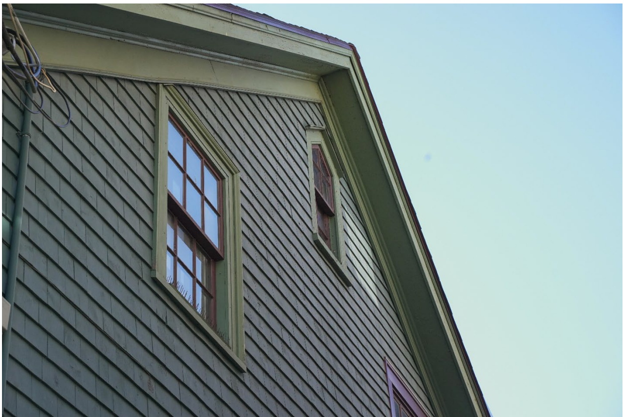
Figure 20: Detail of side windows (Feb. 15, 2023)
