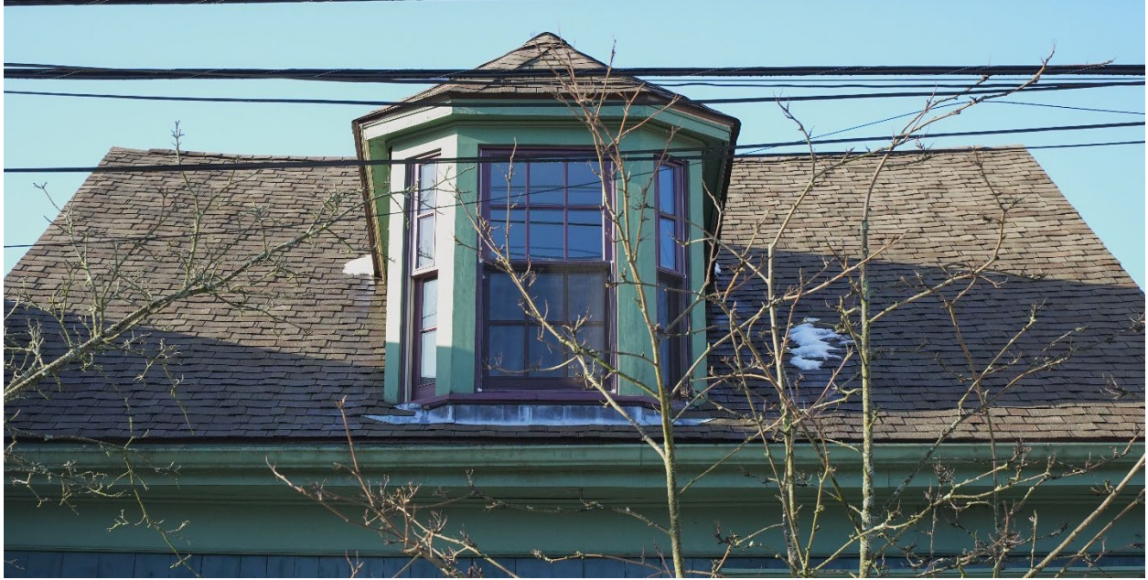
Figure 19: Detail of Scottish dormer (Feb. 15, 2023)
