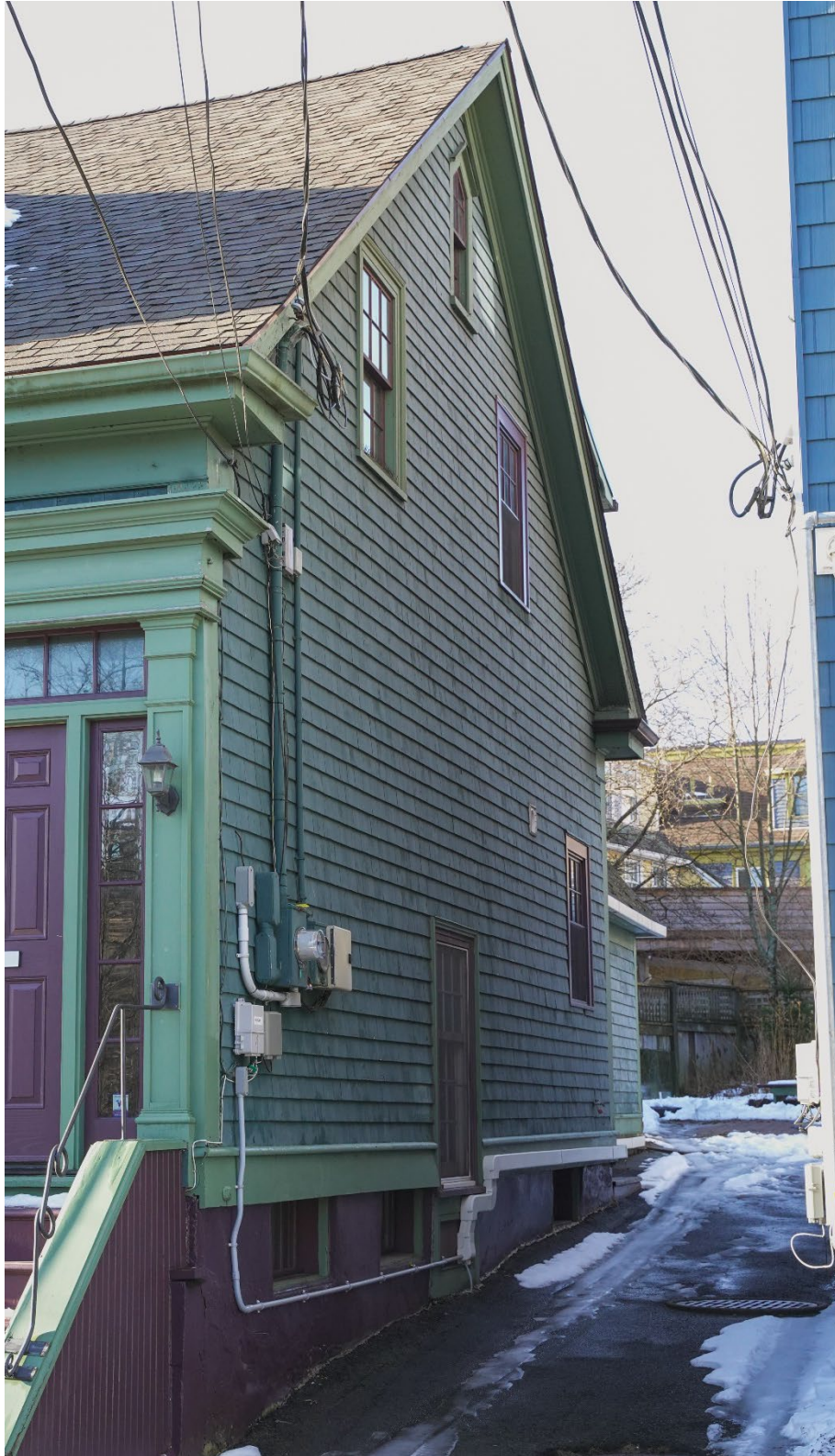
Figure 18: Northern elevation as viewed from the northeast (Feb. 15, 2023)
