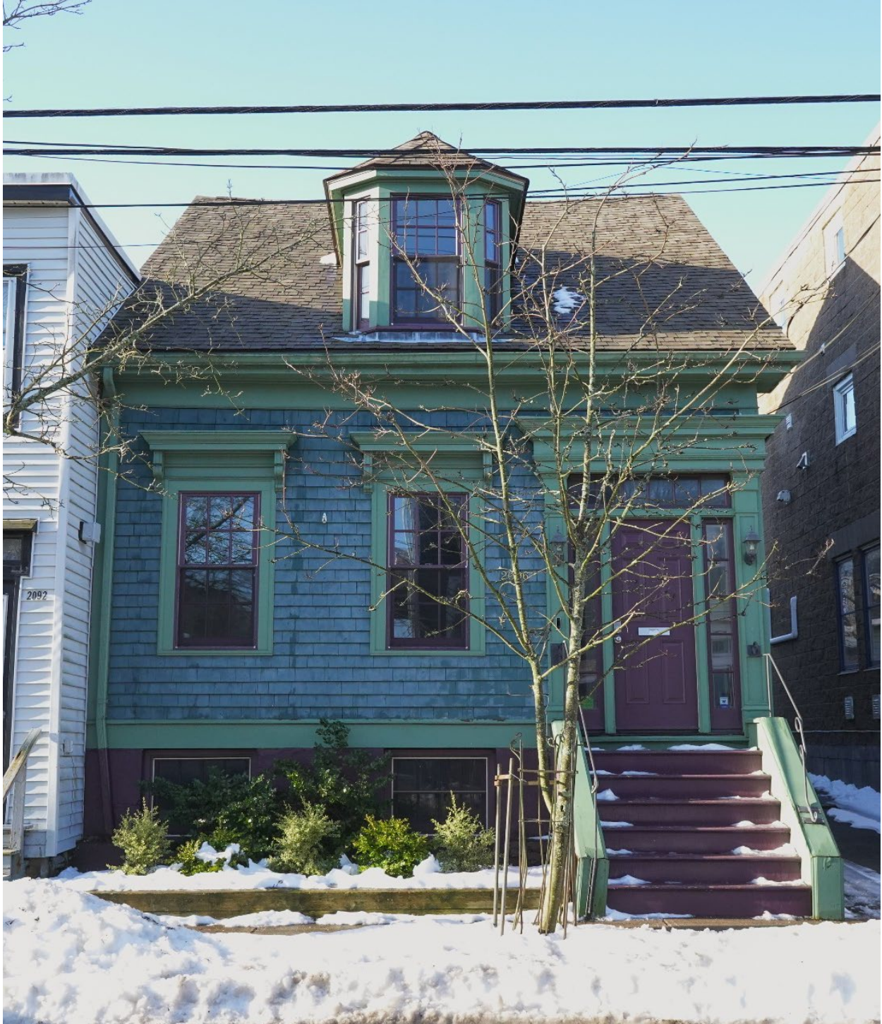
Figure 15: Eastern elevation (Feb. 15, 2023)
