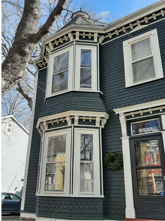
Figure 13: Two-storey Bay window with conical roof and crestring on the north elevation (Staff photo, 22 February 2023)
