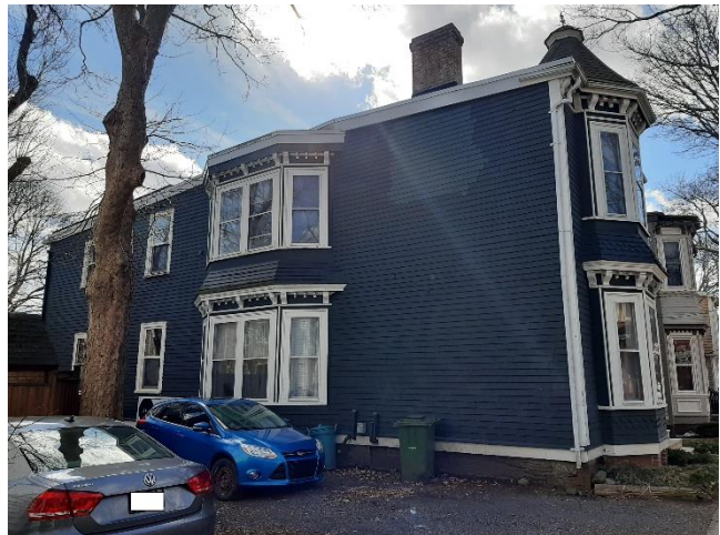
Figure 2: 6032-6034 Charles Street, showing both the north and east two-storey bay windows (Staff photo, 22 February, 2023)
