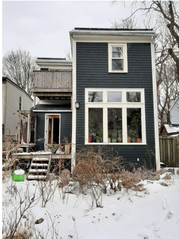
Figure 10: South elevation (Staff photo, 02 March 2023)
