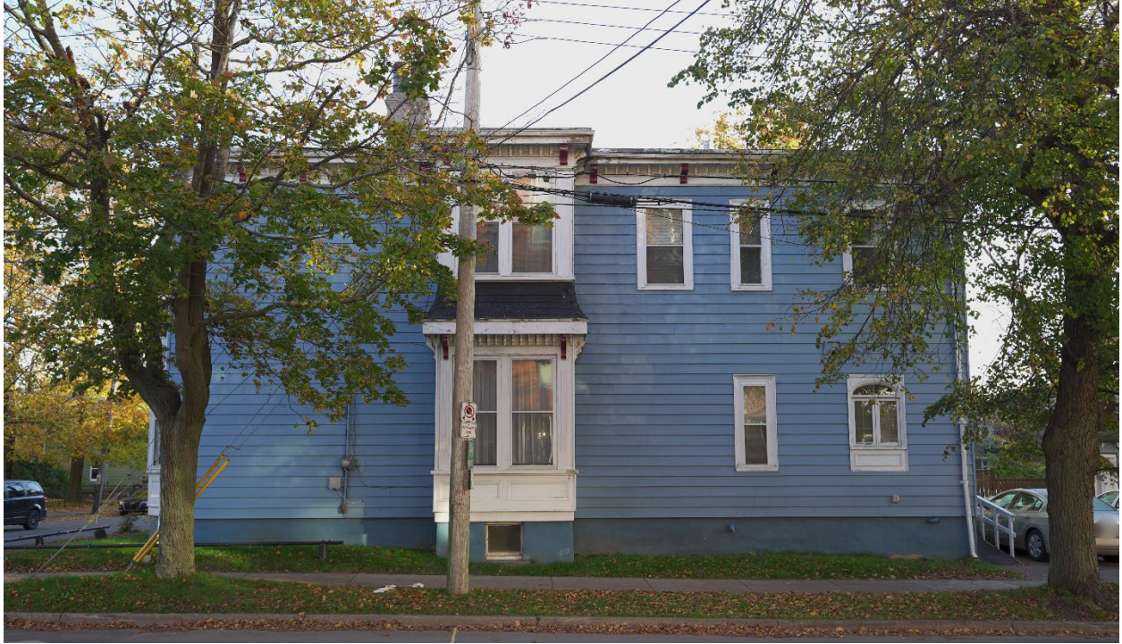
Figure 16: Southwestern elevation (Nov. 4, 2022)
