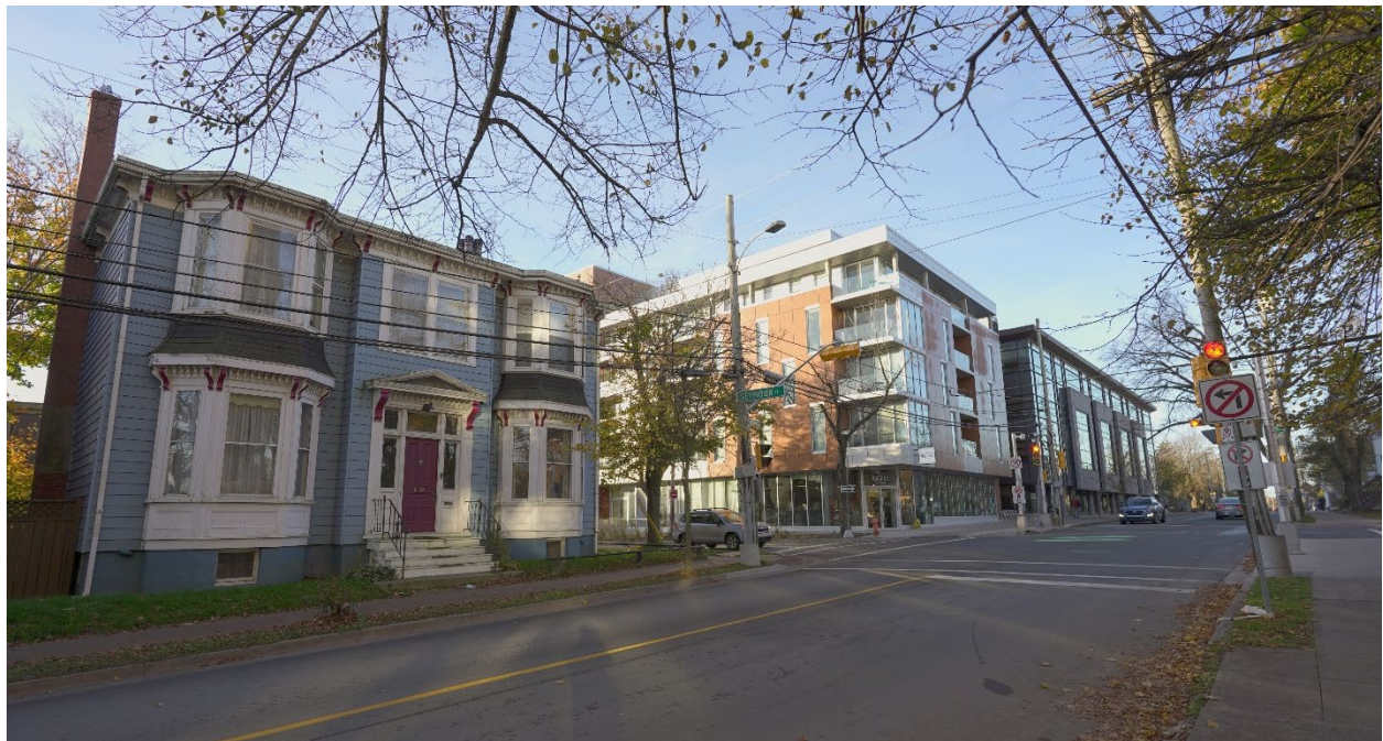
Figure 30: View looking west, with 6112 Coburg Road to the left. (Nov. 4, 2022)
