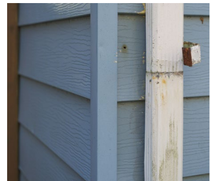
Figure 26: Closeup of aluminum siding (Nov. 4, 2022)
