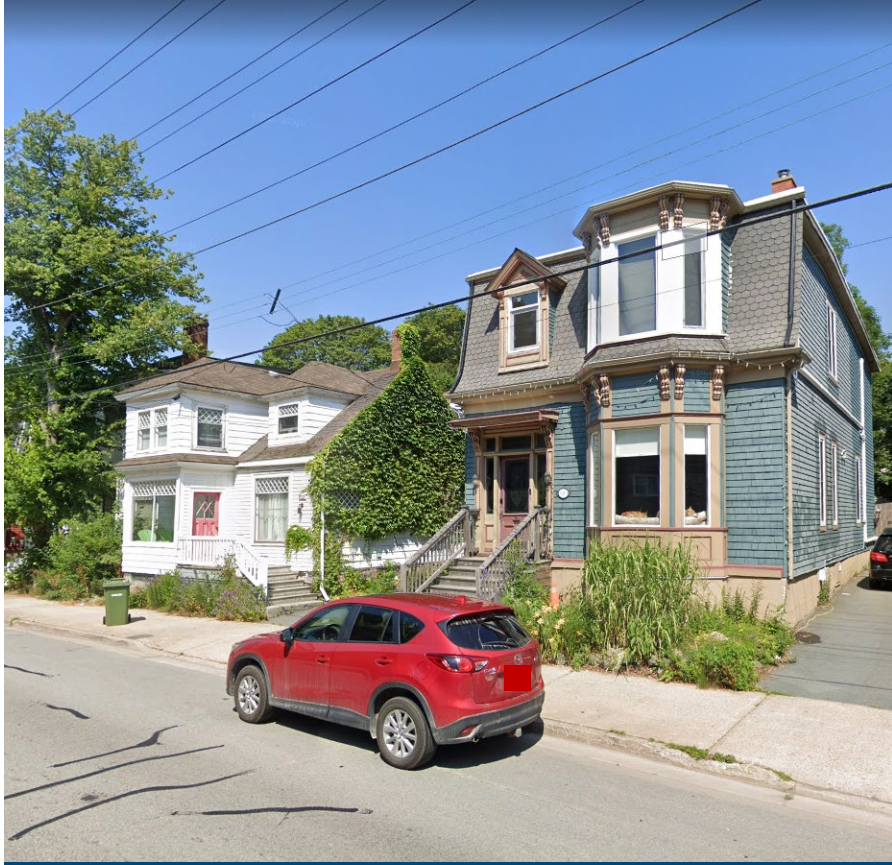
Nearby registered properties: Hartshorne-Lownds House [left] and Toomey House [right]
