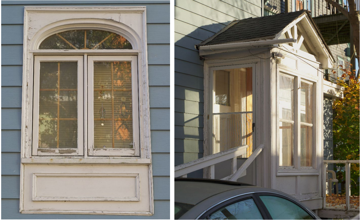
Figure 24: Detail of side window and rear porch (Nov. 4, 2022)
