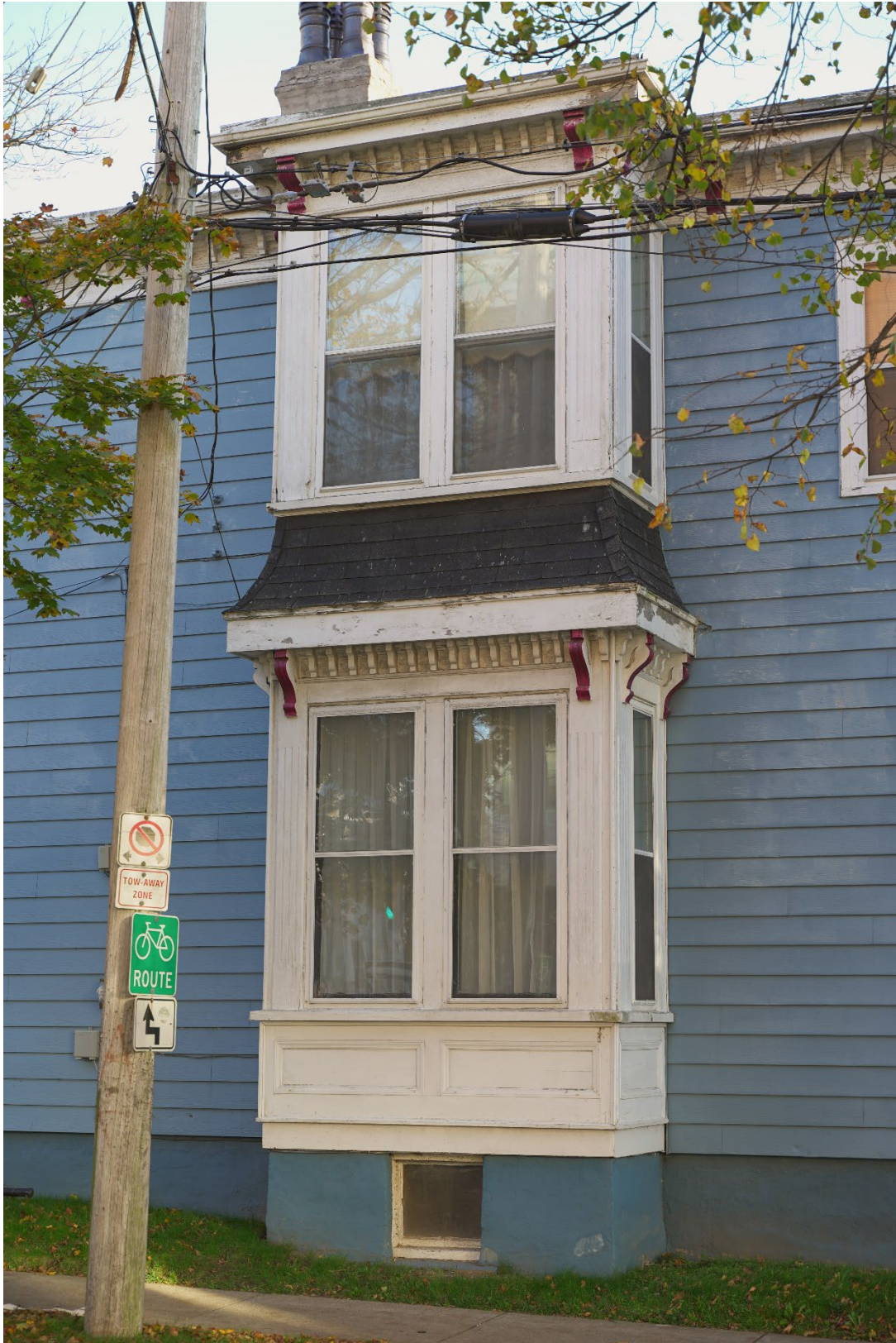
Figure 23: Detail of side bay (Nov. 4, 2022)
