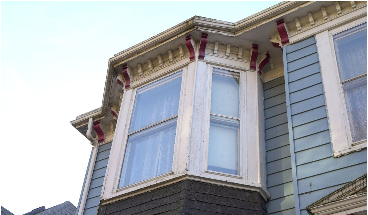
Figure 22: Detail of upper bay (Nov. 4, 2022)
