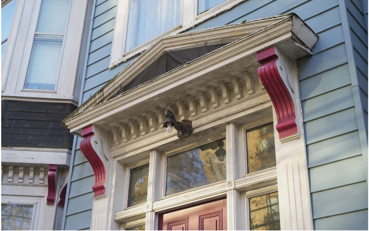
Figure 21: Detail of front porch (Nov. 4, 2022)
