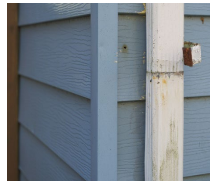
Figure 26: Closeup of aluminum siding (Nov. 4, 2022)
