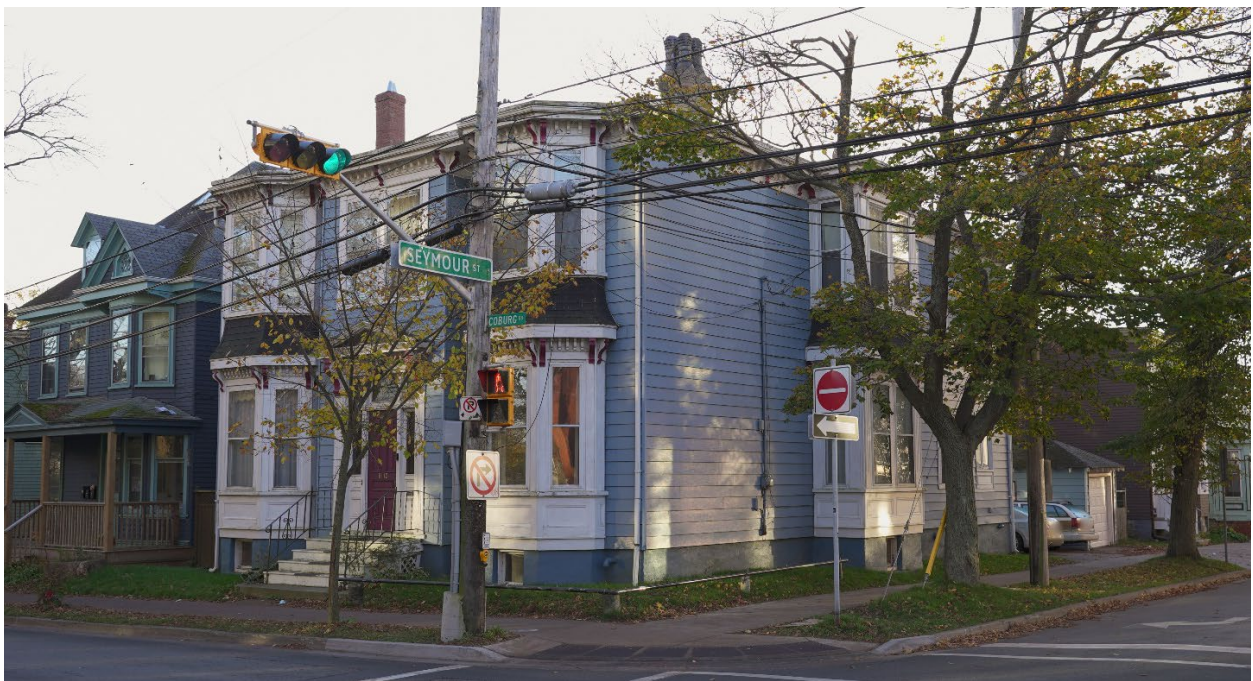
Figure 15: Southeastern elevation (Nov. 4, 2022)
