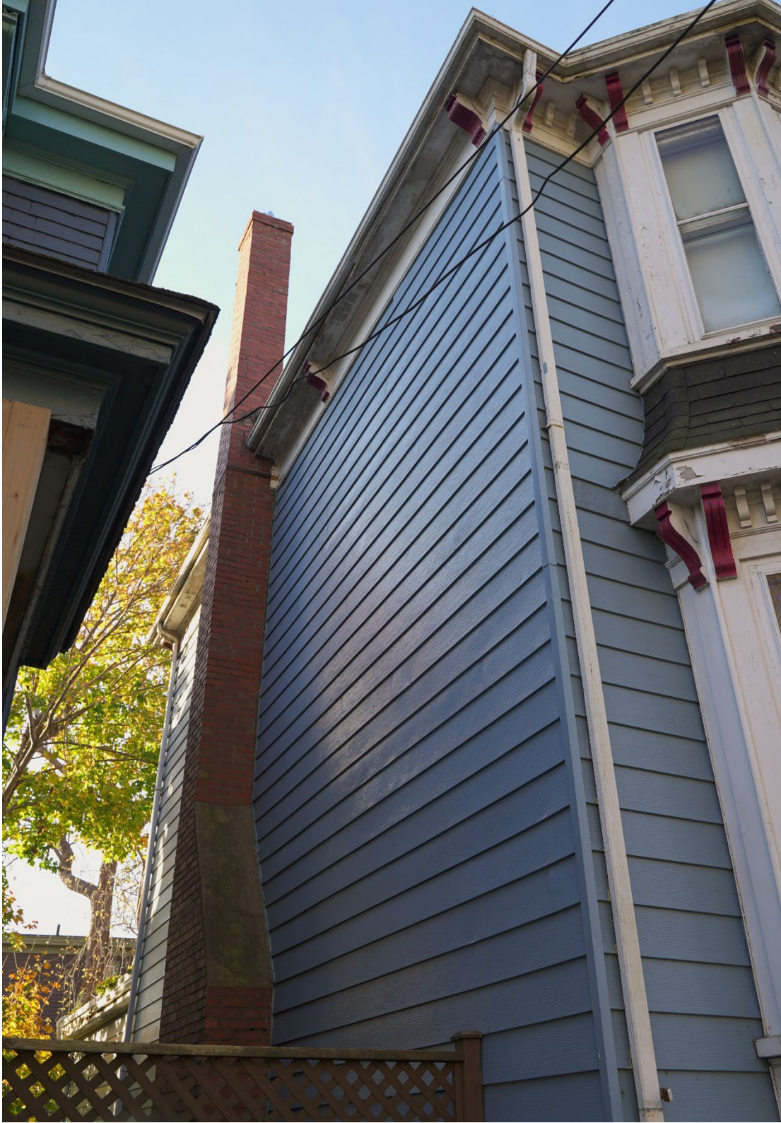
Figure 18: Eastern elevation (Nov. 4, 2022)
