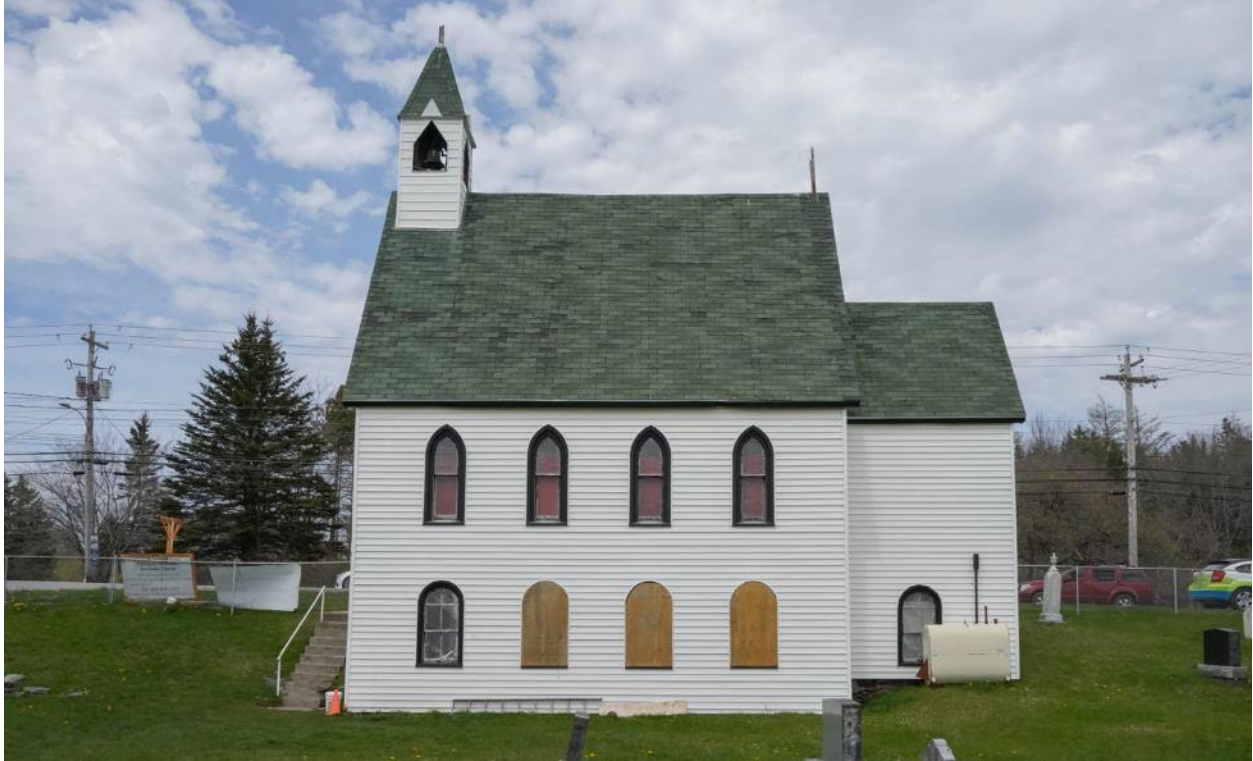
Figure 23: View of the southern elevation (May 13, 2022)
