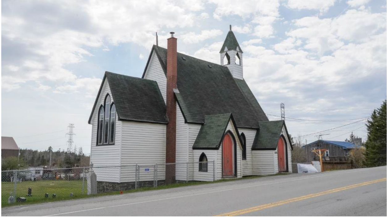
Figure 19: View of the southeast elevation (May 13, 2022)
