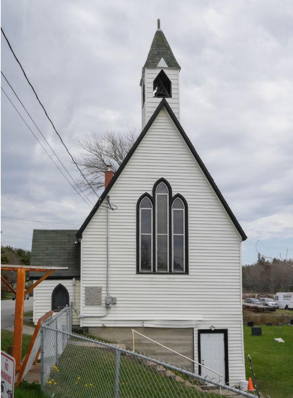
Figure 21: View of the western elevation (May 13, 2022)
