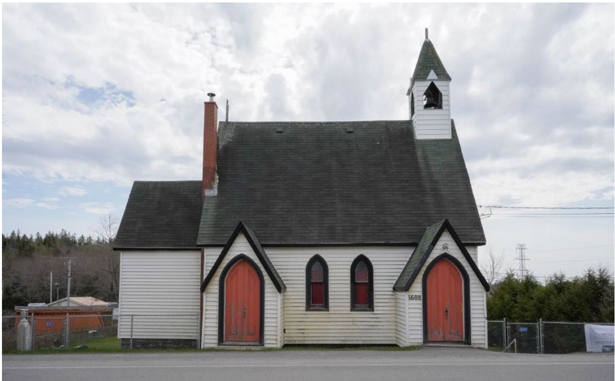
Figure 20: View of the northern elevation (May 13, 2022)
