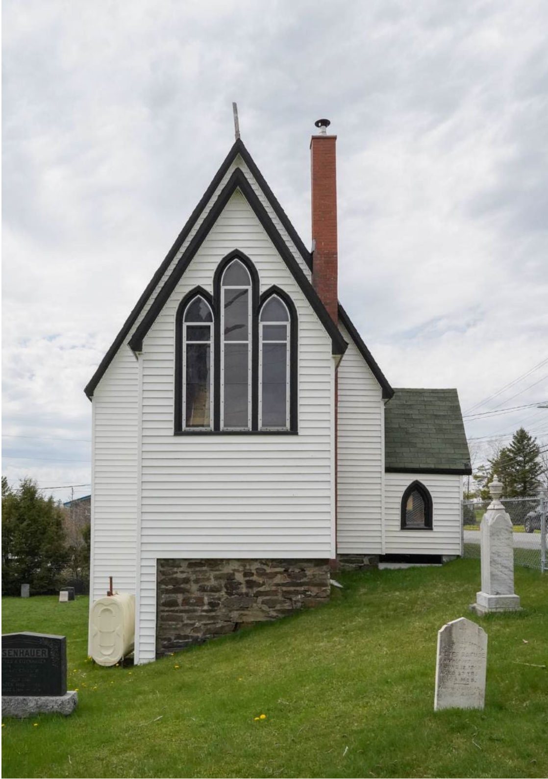
Figure 22: View of the eastern elevation (May 13, 2022)
