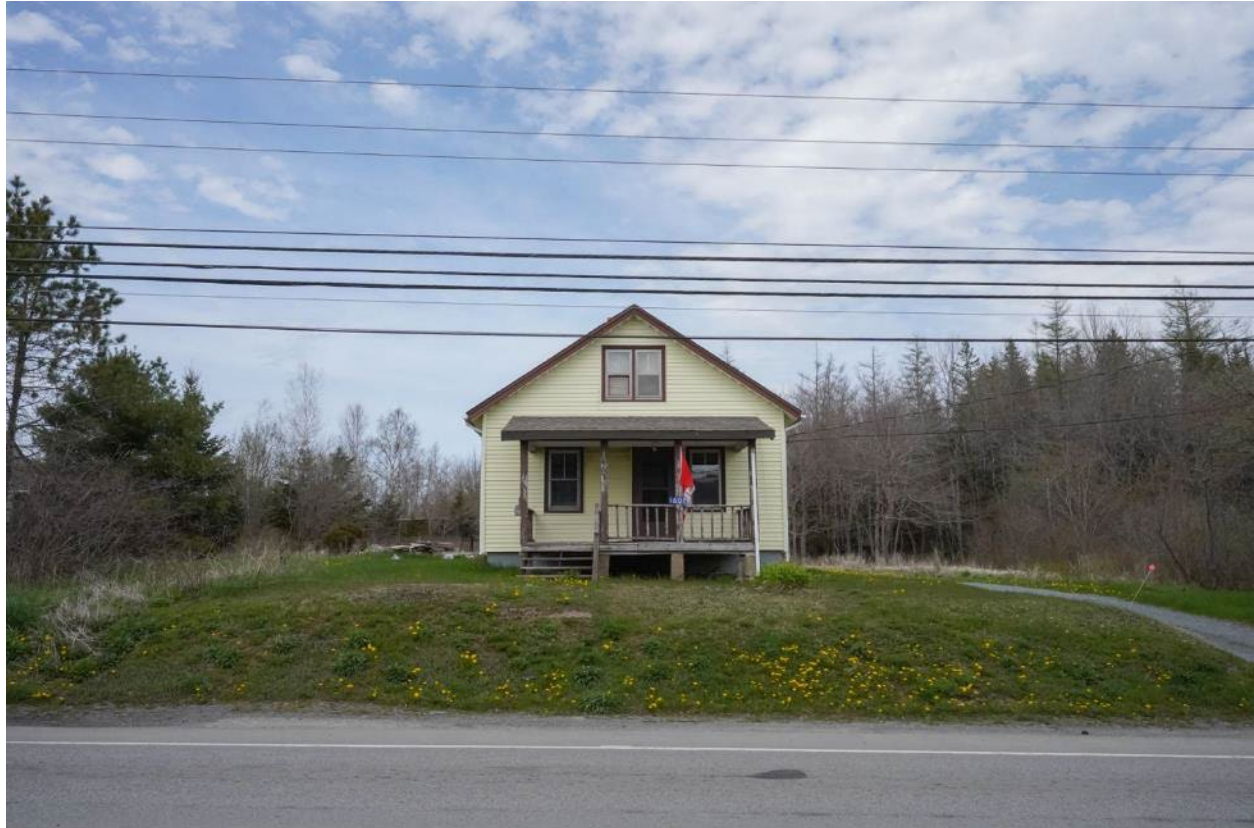
Figure 27: View looking north across Hammonds Plains Road from St. Nicholas, showing the former Orman Roman [later Margaret Grandy] house. (May 13, 2022)
