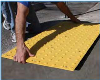
*Fast, easy installation with included adhesive and anchor system. Apply adhesive to scored areas on back, place in desired location and install anchors*
