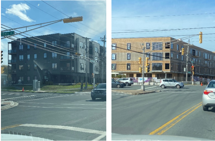
New Multi-Unit Buildings in Lower Sackville
