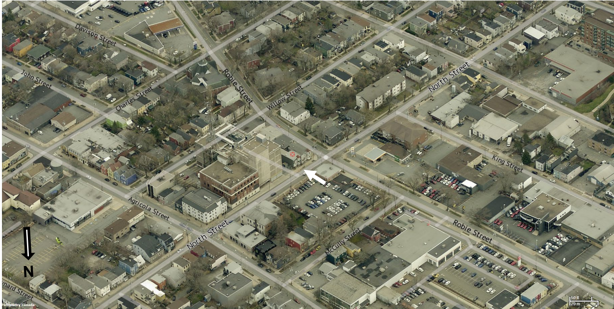
Figure 26: Aerial pictometry image looking south with 5812-5814 North Street highlighted by an arrow. (April 12, 2022)
