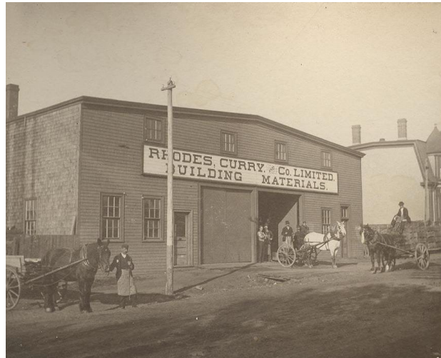
Figure 16: Photograph of the Halifax branch of Rhodes, Curry & Co. Ltd. situated at [then] 300-302 Robie Street. 52
