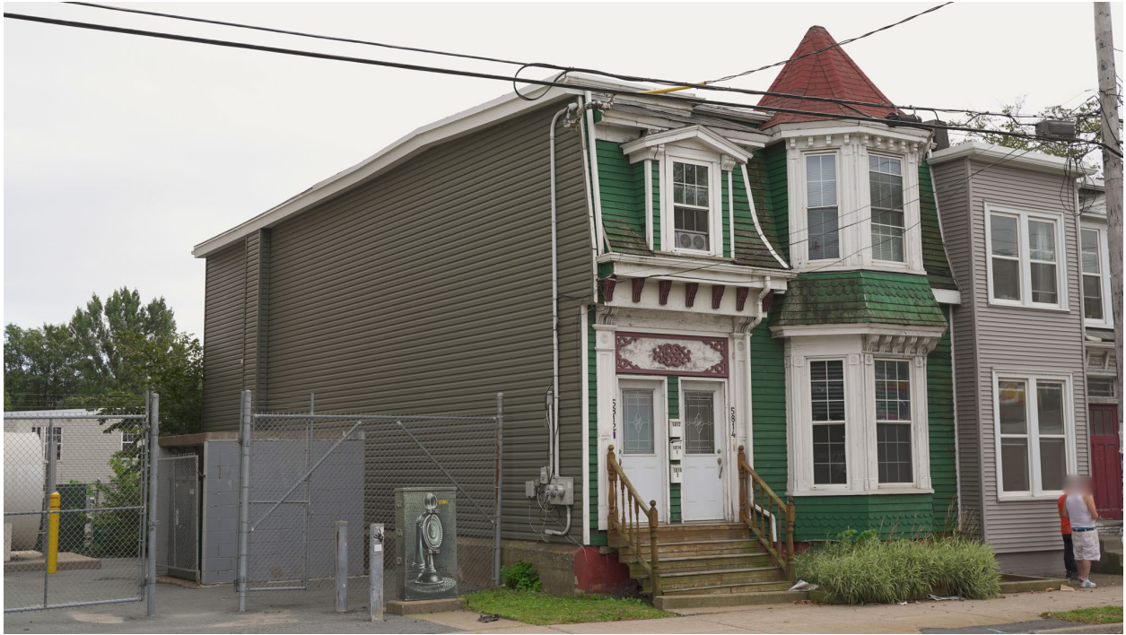
Figure 18: Northeastern elevation (August 31, 2022)
