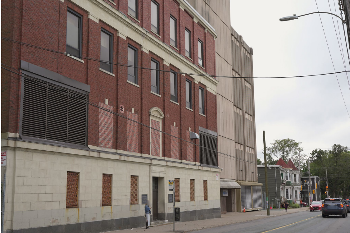
Figure 29: The red-brick former Maritime Telegraph and Telephone Co. building in the foreground with the subject property visible in the background [unregistered, contributing heritage]. (August 31, 2022)
