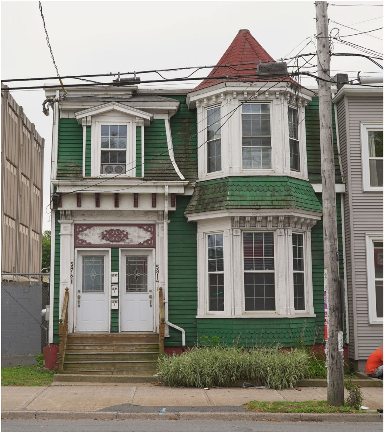
Figure 17: Northern elevation (Aug 31, 2022)
