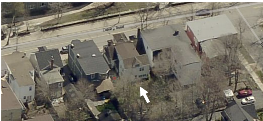
Figure 41: Aerial pictometry showing the rear of 6221 Coburg Road and its additions. (May 6, 2020)
