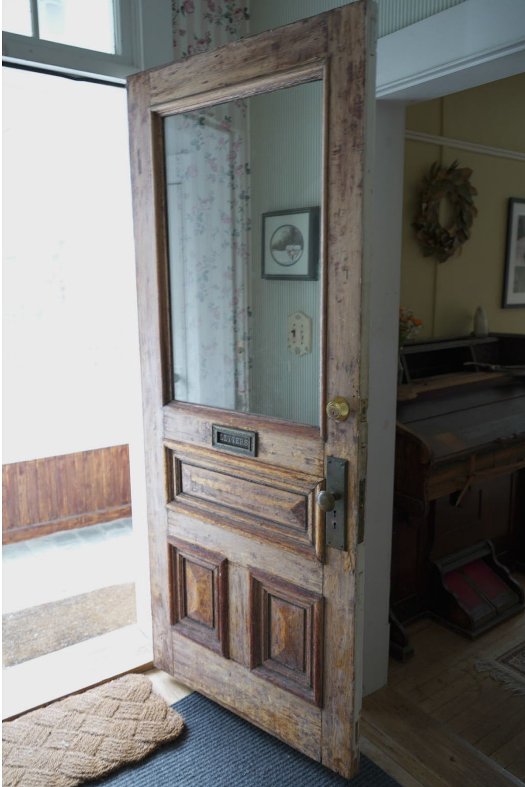
Figure 37: Detail of front door (October 24, 2022)
