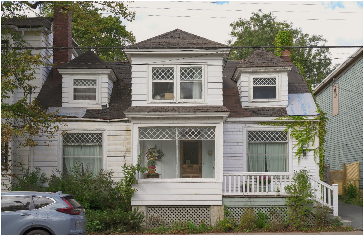
Figure 30: Southern elevation (August 31, 2022)
