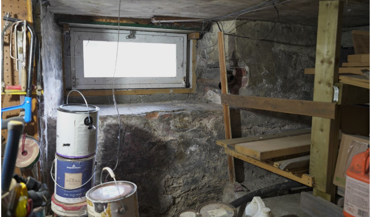
Figure 25: Photo showing thickness of the foundation. (October 24, 2022)
