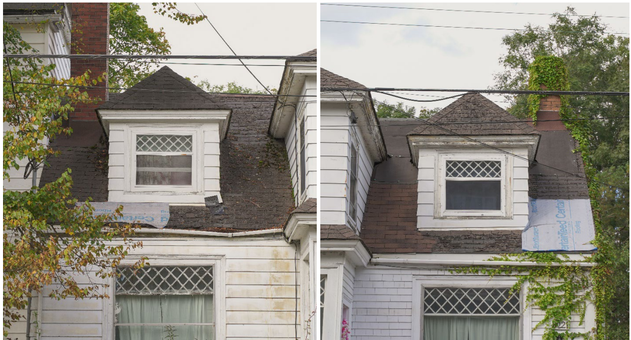
Figure 36: Detail of the dormers (August 31, 2022)
