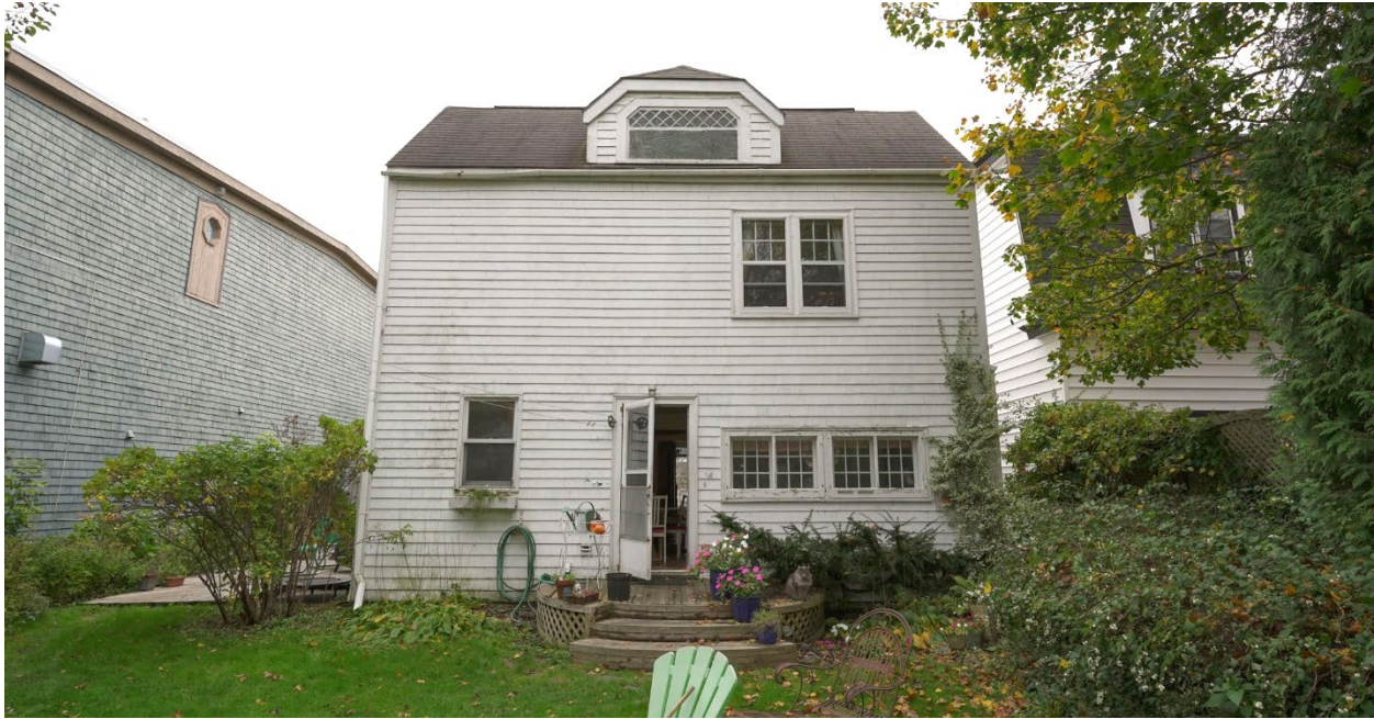
Figure 33: Northern elevation (October 24, 2022)
