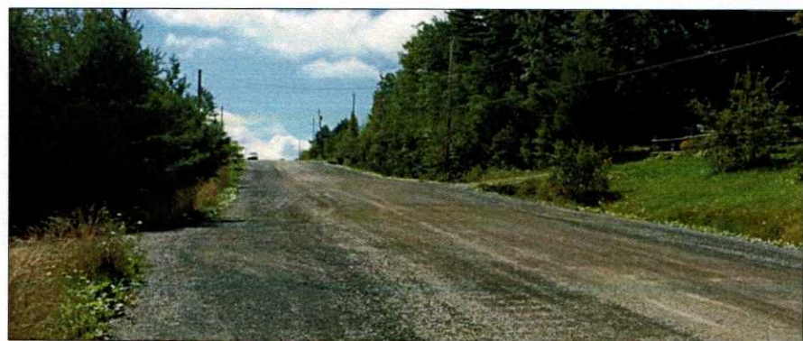
Photo 6: Looking south (to the left) on Trinity Lane from the proposed north site access Intersection
