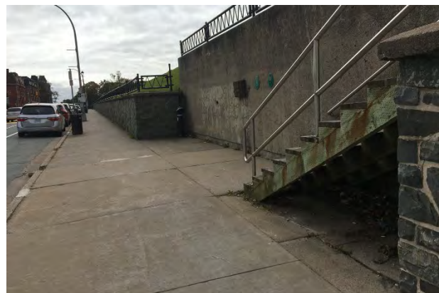
Figure 3 -Brunswick Streetscape at Base of Clocktower
