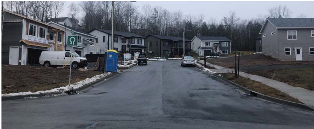
Photo 2 - Splinter Court from Daisy Drive
