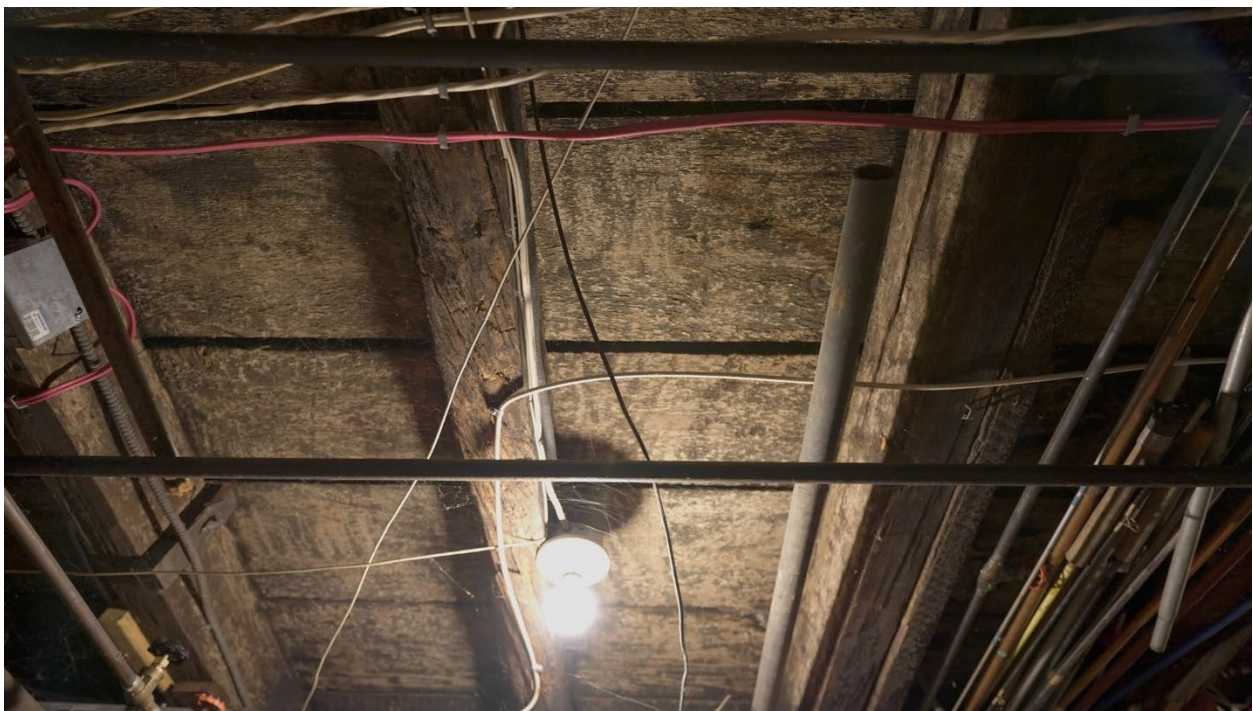
Figure 26: Photo showing subfloor and joist structure. (October 24, 2022)
