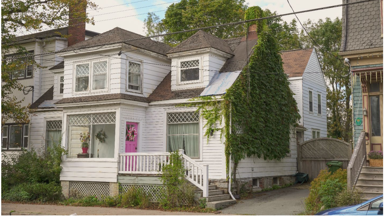
Figure 31: Southeastern elevation (August 31, 2022)
