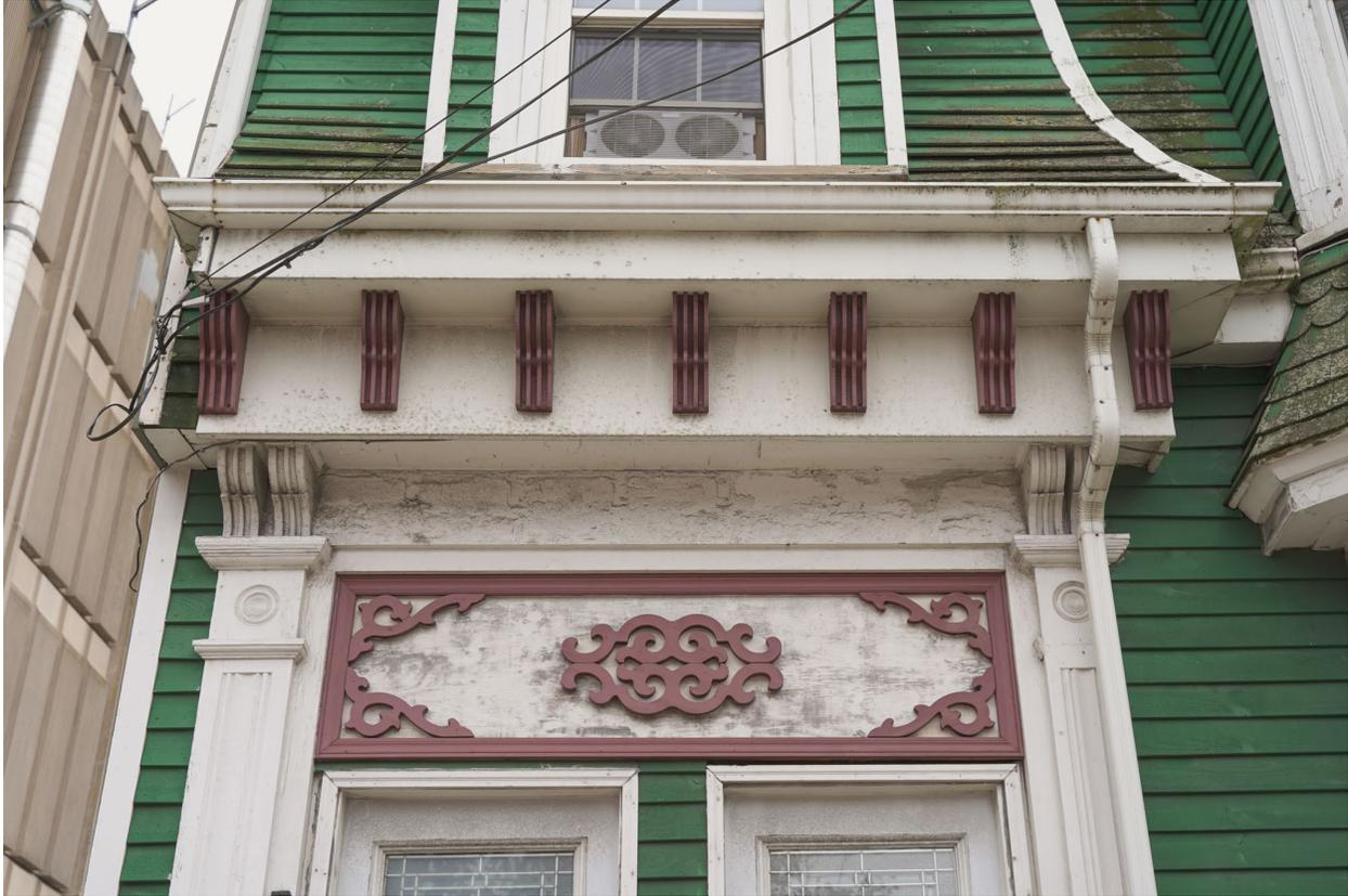
Figure 22: Detail of double cornice, pilasters, and missing transom (August 31, 2022)
