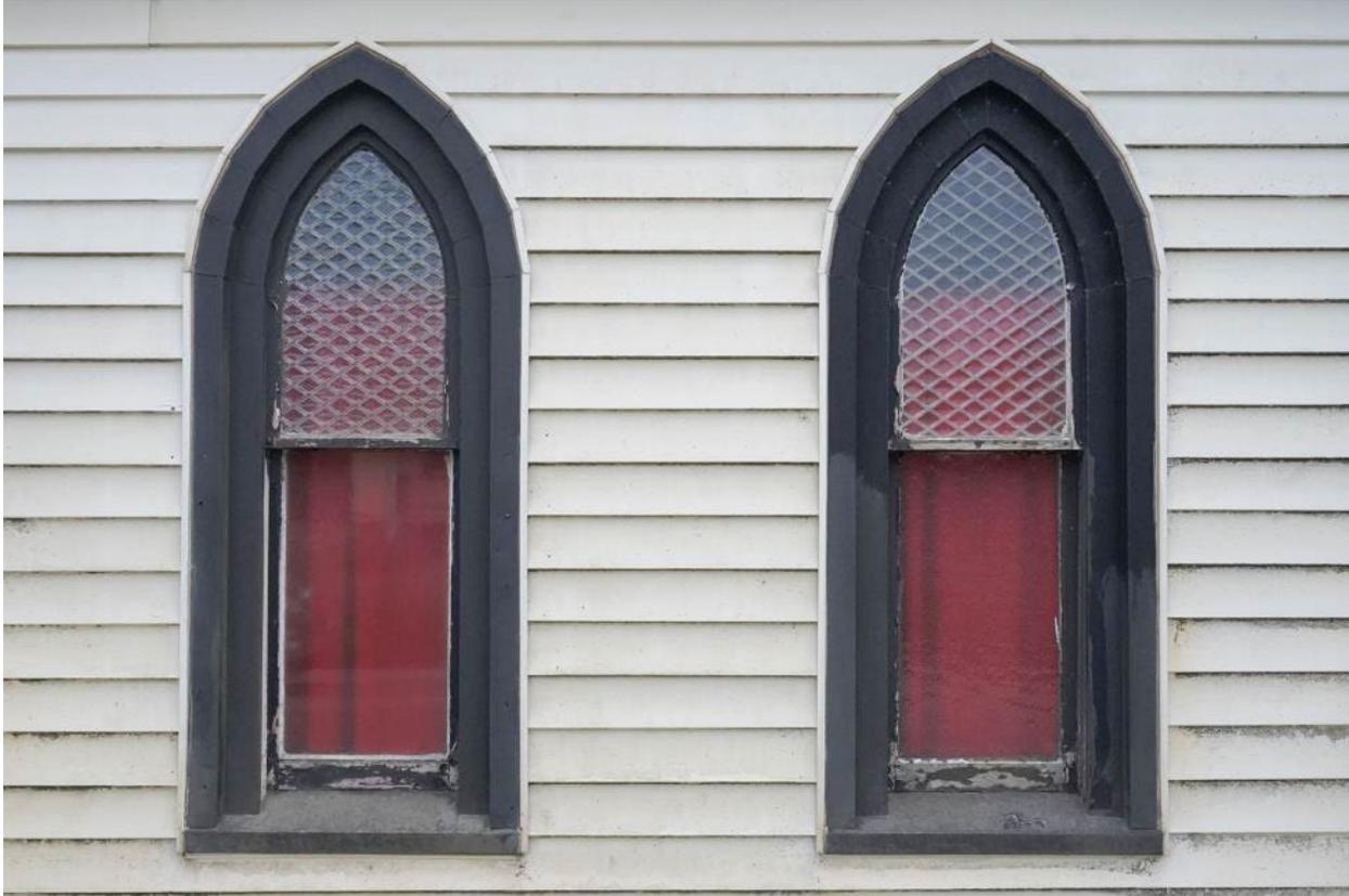
Figure 18: Two windows on the northern elevation, with upper sashes made of rolled white cathedral glass with a longitudinal diamond pattern similar to the pattern known as “quarry rolled”.(May 13, 2022)
