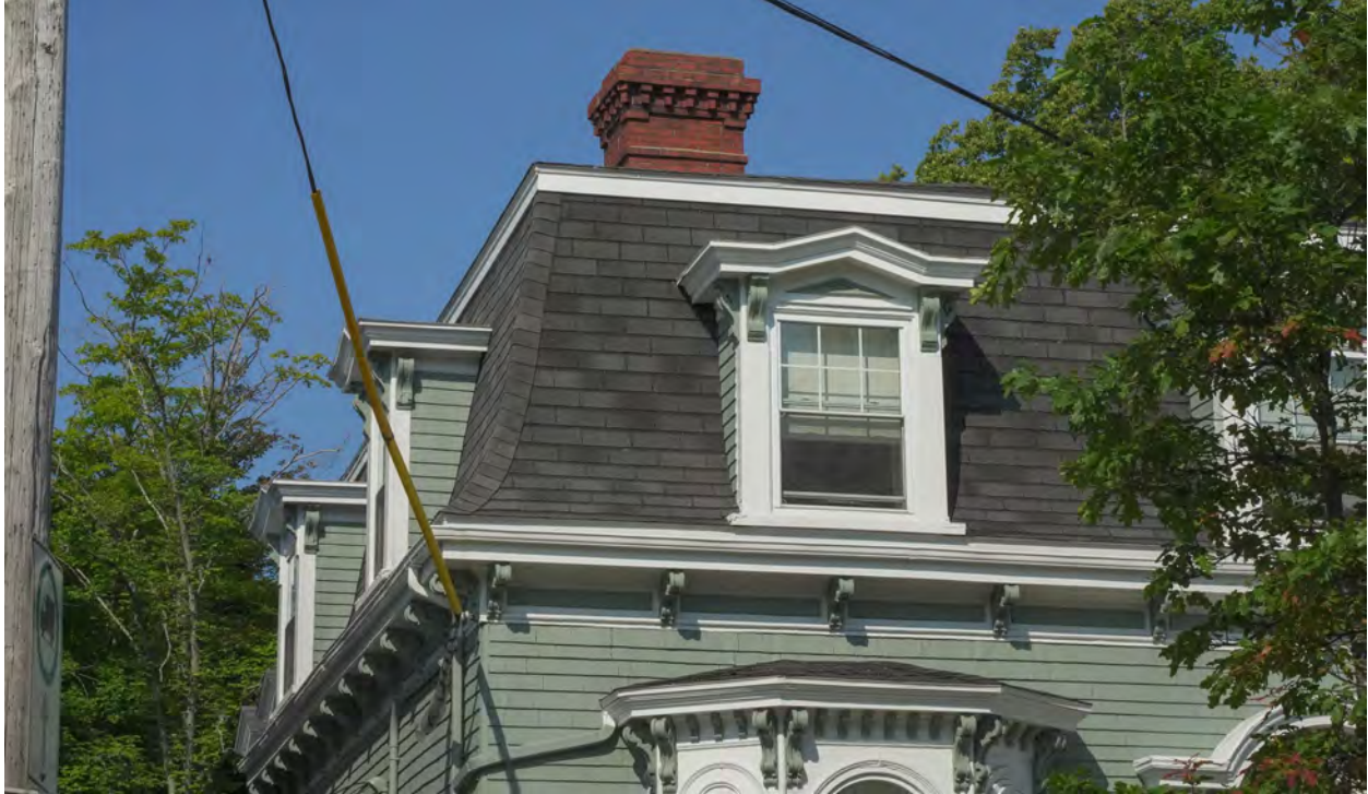
Figure 19: Detail of the dormers cornice and chimney (July 21, 2022)
