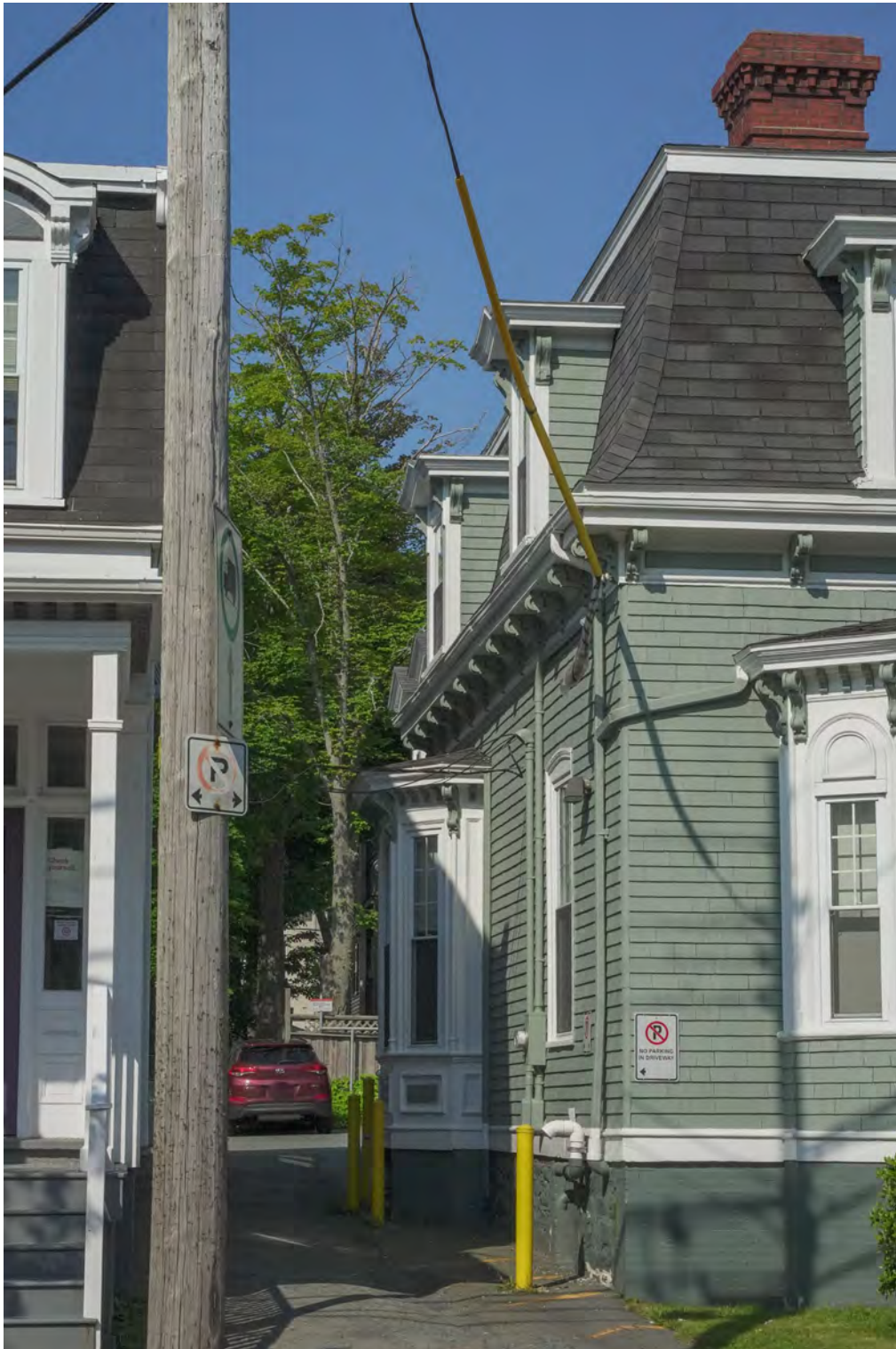
Figure 17: Southern elevation as viewed from the east (July 21, 2022)
