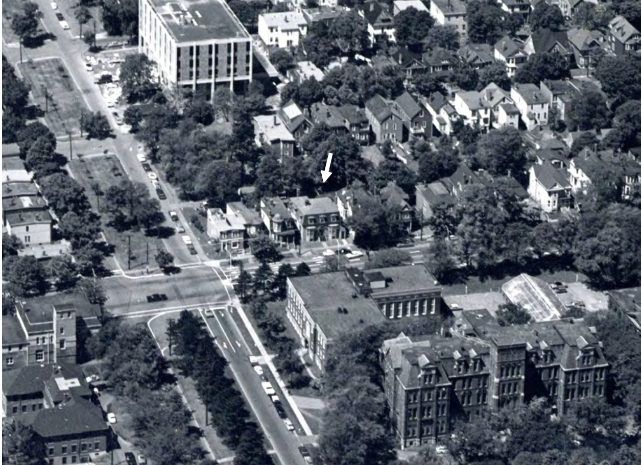
Figure 6: 1322 Robie Street as shown in an aerial photo of Dalhousie dating between 1957 and 1970. 5
