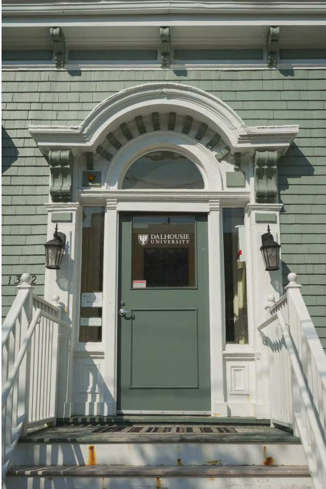
Figure 23: Detail of the front door, transom, & sidelights (July 21, 2022)
