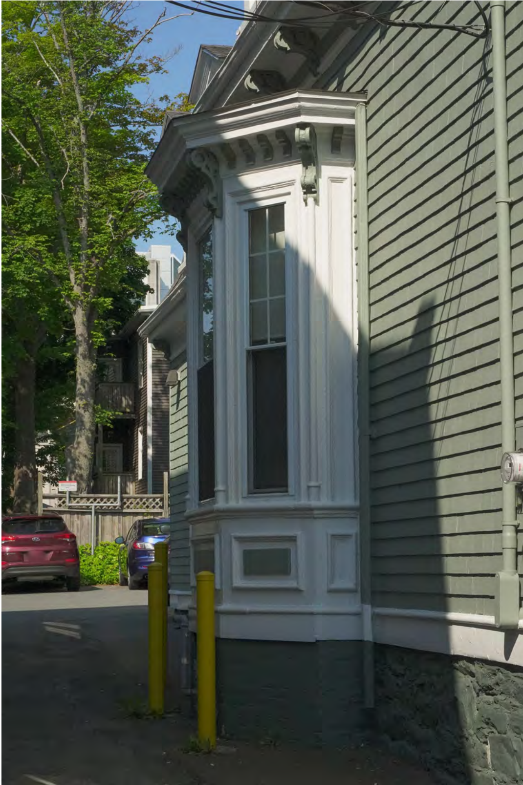
Figure 22: Detail of the southern side bay window with cornice, mouldings, and panelling (July 21, 2022).
