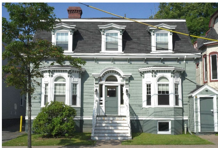
Figure 1: Western elevation of 1322 Robie Street in July 2022
