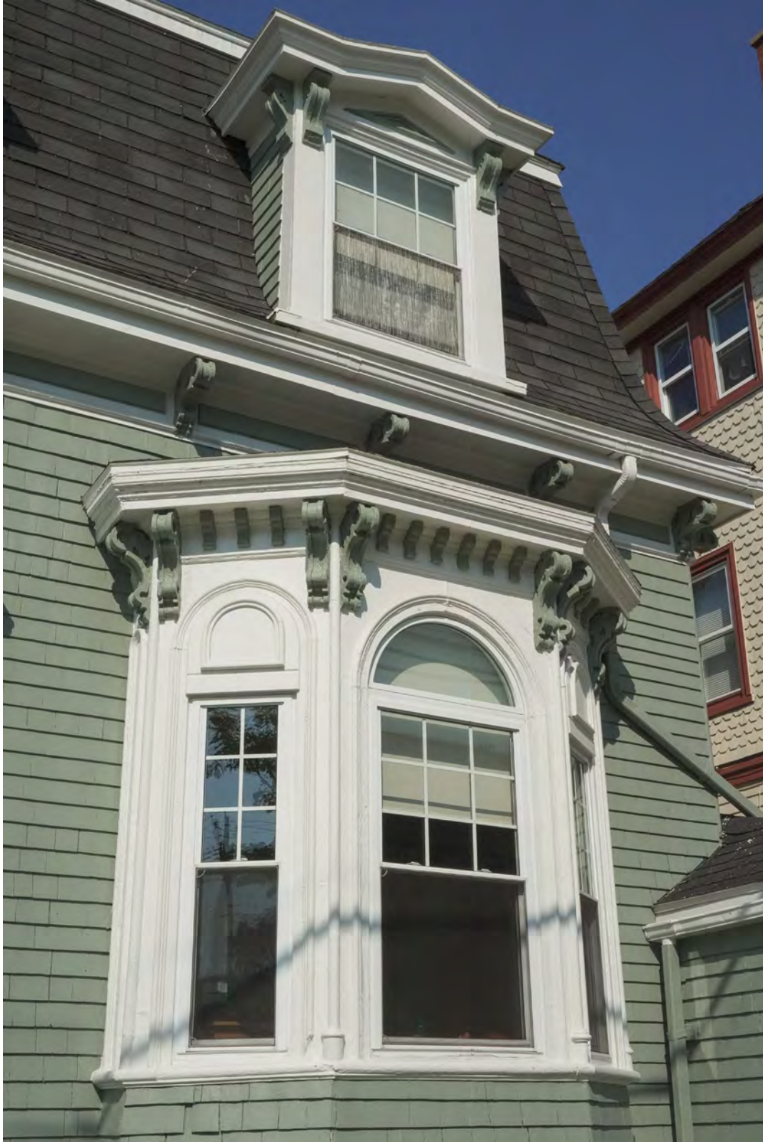
Figure 21: Detail of the front right bay window with details and cornice (July 21, 2022).
