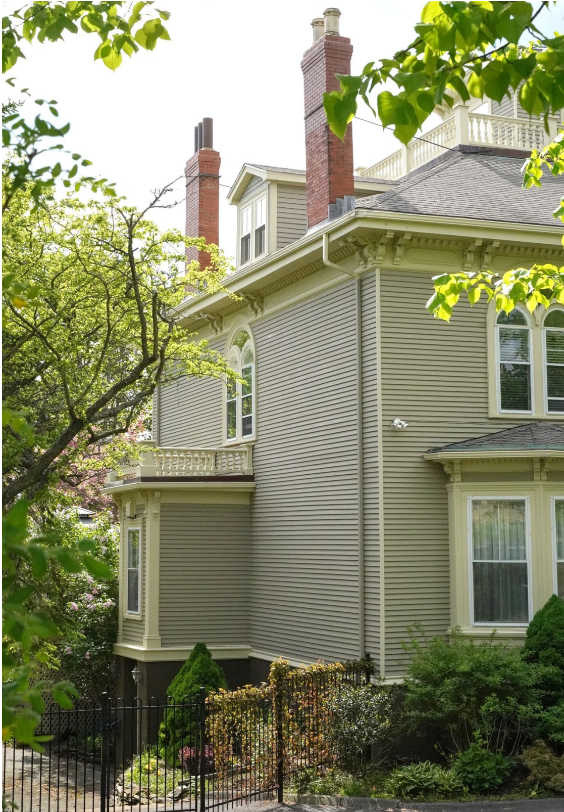
Figure 19: Southern elevation as viewed from the southeast (May 30, 2022)
