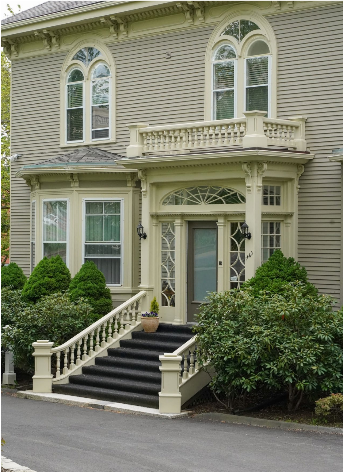
Figure 20: Detail view of the front porch (May 30, 2022)
