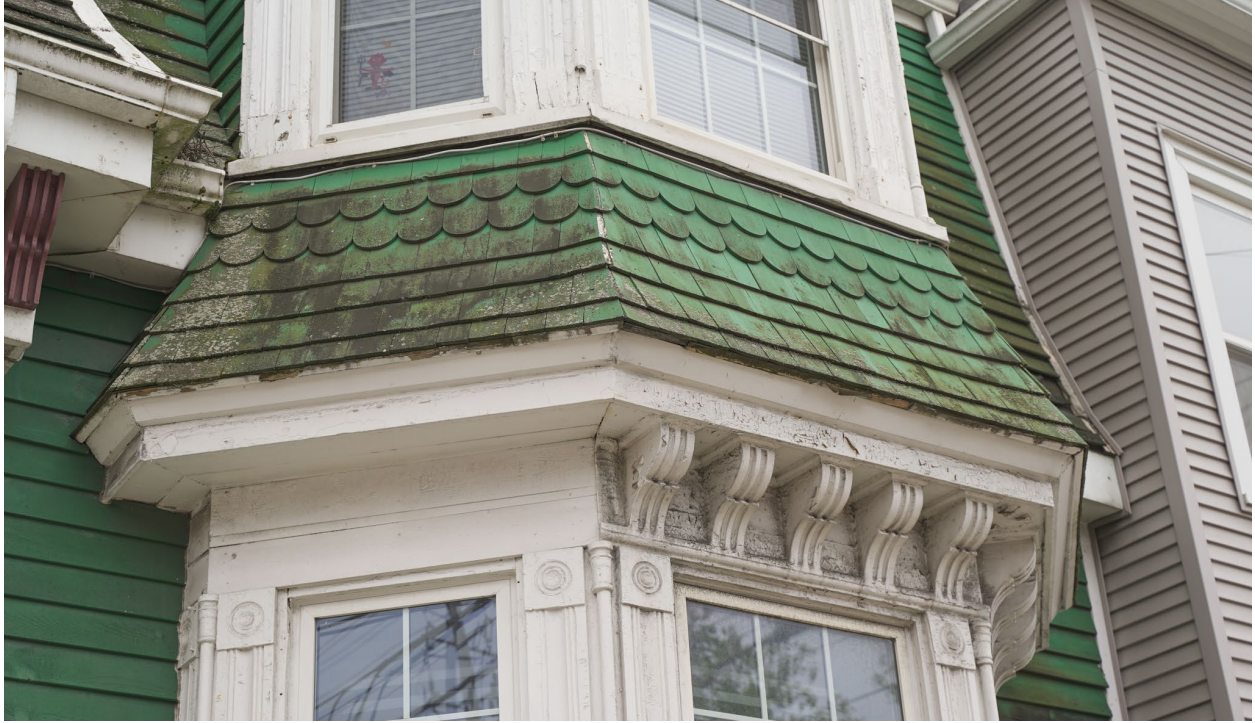
Figure 20: Detail of bay window (August 31, 2022)
