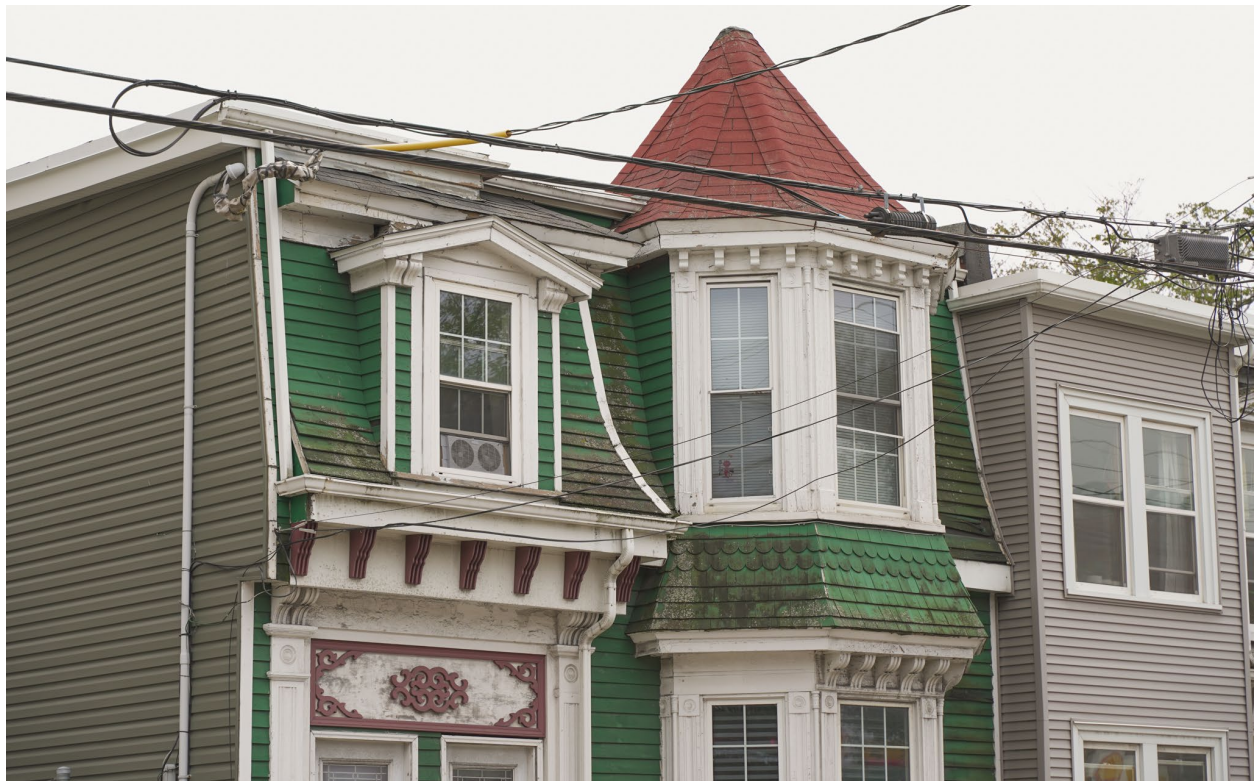
Figure 19: Detail of upper storey (August 31, 2022)
