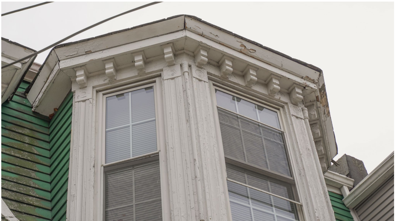
Figure 21: Detail of bay window (August 31, 2022)
