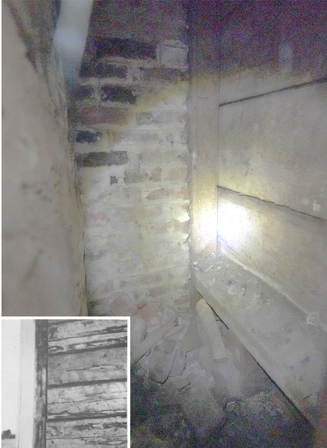
Figure 29: View of the internal construction the subject property's western wall, showing what appears to be either squared-logs or thick-sawn planks slotted into channels in the vertical posts of the house's frame [a technique known as poteaux et pièce coulissante] and the western brick chimney. (October 24, 2022) At bottom-left is an inset photo showing an example of "poteaux-en-coulisse" wall construction.
