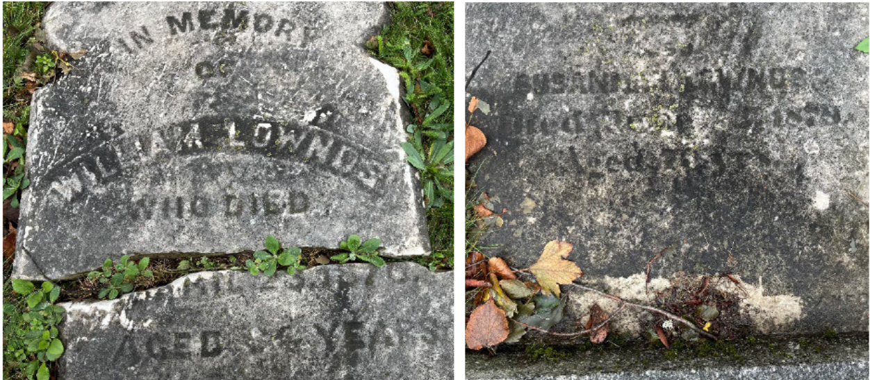
Figure 20: A pair of photos showing the top [left] and bottom [right] of a damaged gravestone at Camp Hill Cemetery marking the graves of both William Lownds and his sister Susannah Lownds. (September 28, 2022)
