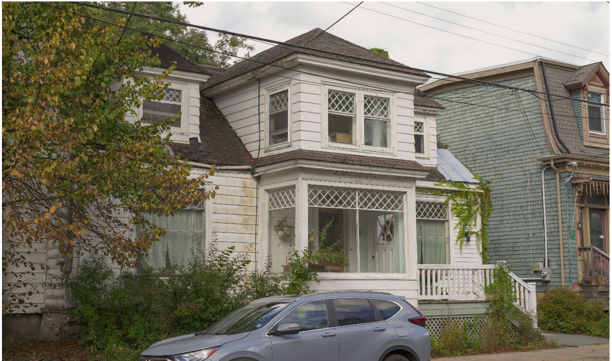
Figure 32: Southwestern elevation (August 31, 2022)
