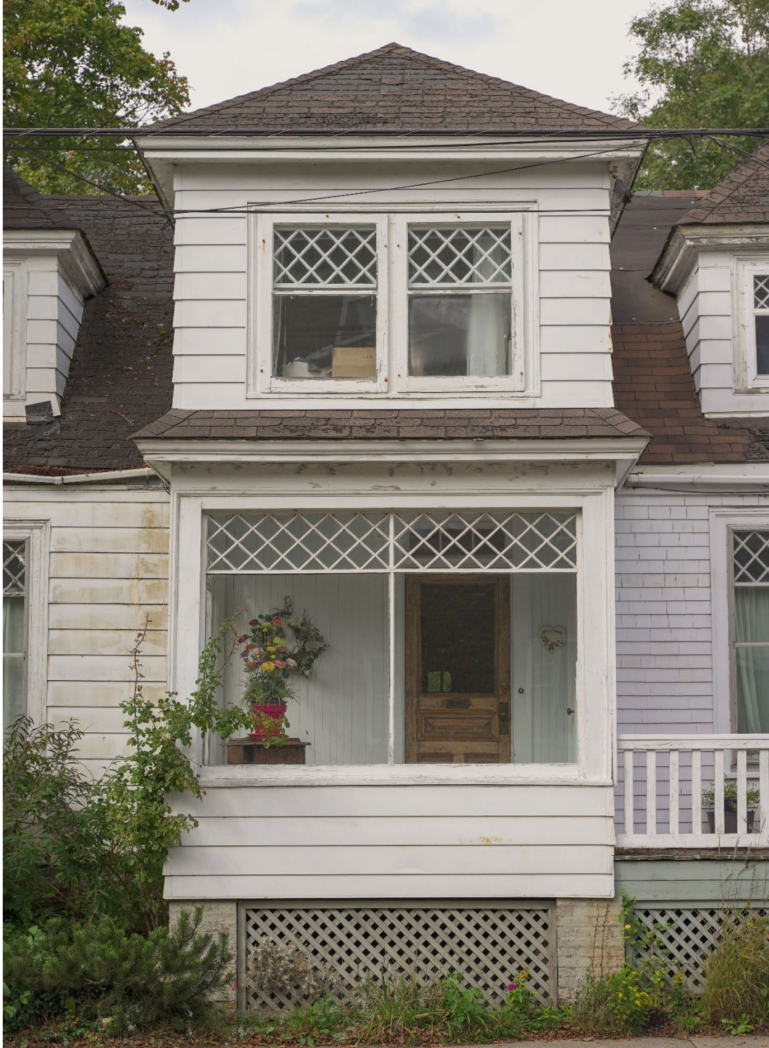
Figure 38: Detail of front porch (September 29, 2022)
