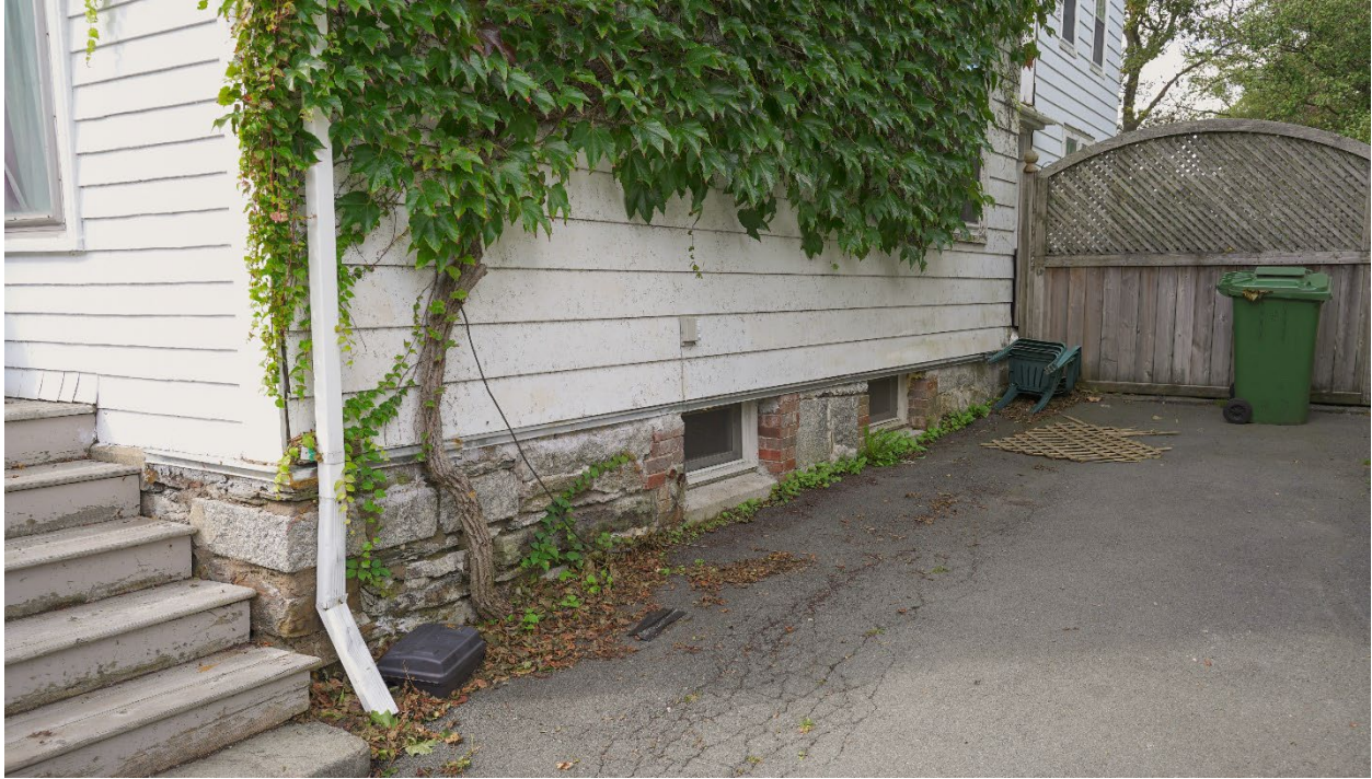
Figure 35: Detail of the foundation (August 31, 2022)
