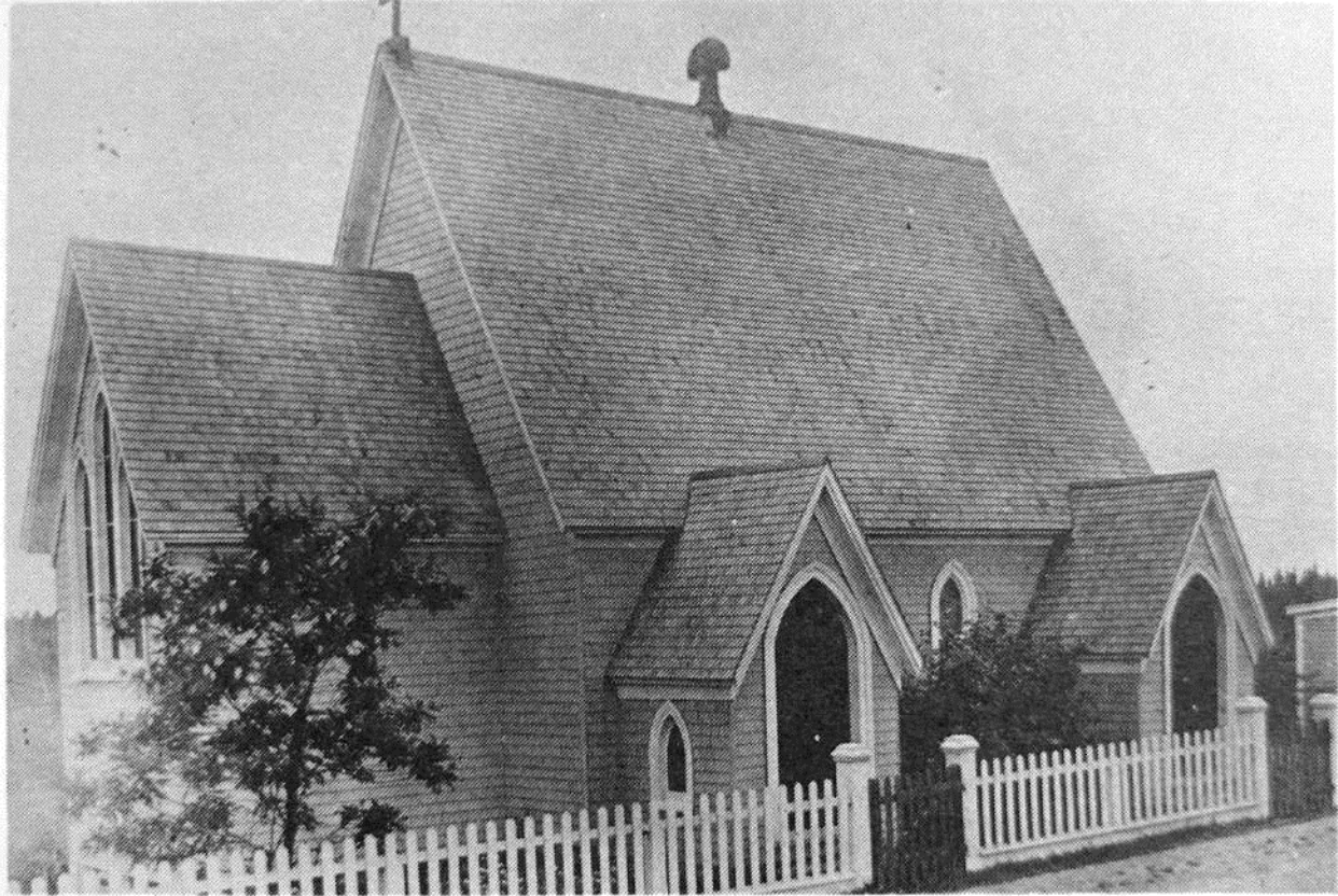
Figure 4: Earliest known photo of St. Nicholas Church, taken pre-1937. Note the lack of steeple, which was a later addition, and the presence of a chimney for the centrally located wood-burning stove, which was later replaced with a furnace and brick chimney.(Evans, 1993)
