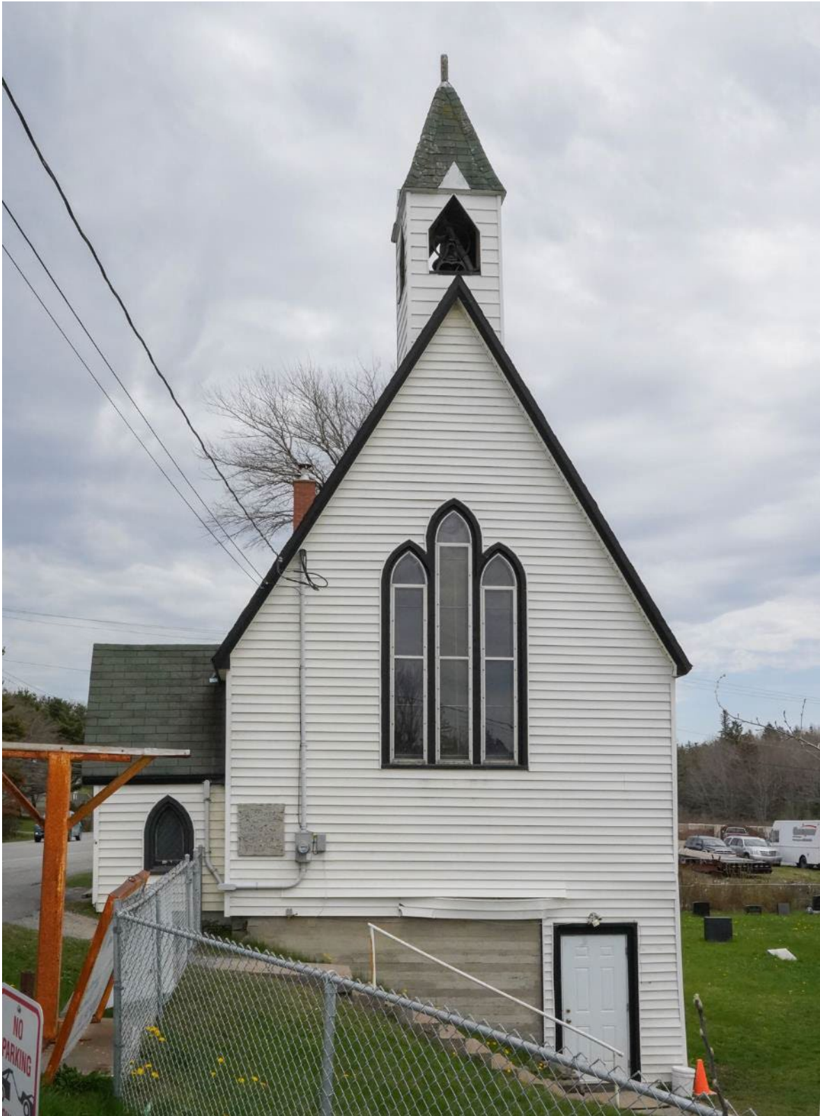
Figure 21: View of the western elevation (May 13, 2022)
