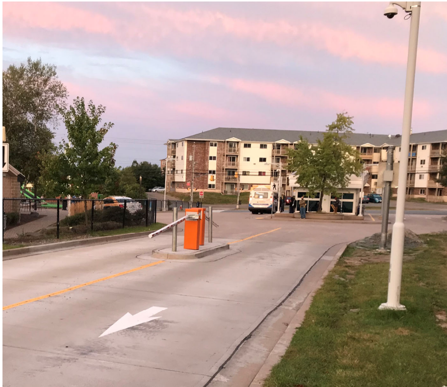
Highfield Terminal Access Gates
