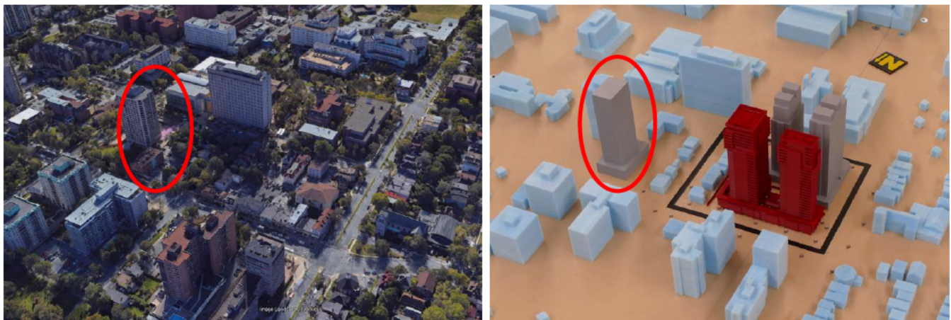
Figure 1: Aerial View of Existing Site (Google Earth™) (Left) and Photograph of Wind Tunnel Study Model – Proposed Configuration (Right)
