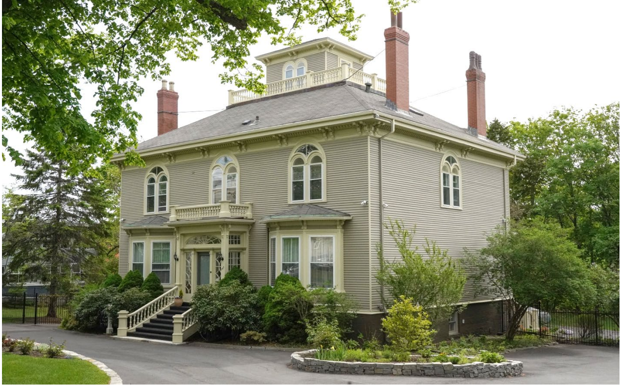
Figure 16: Northeast elevation (May 30, 2022)
