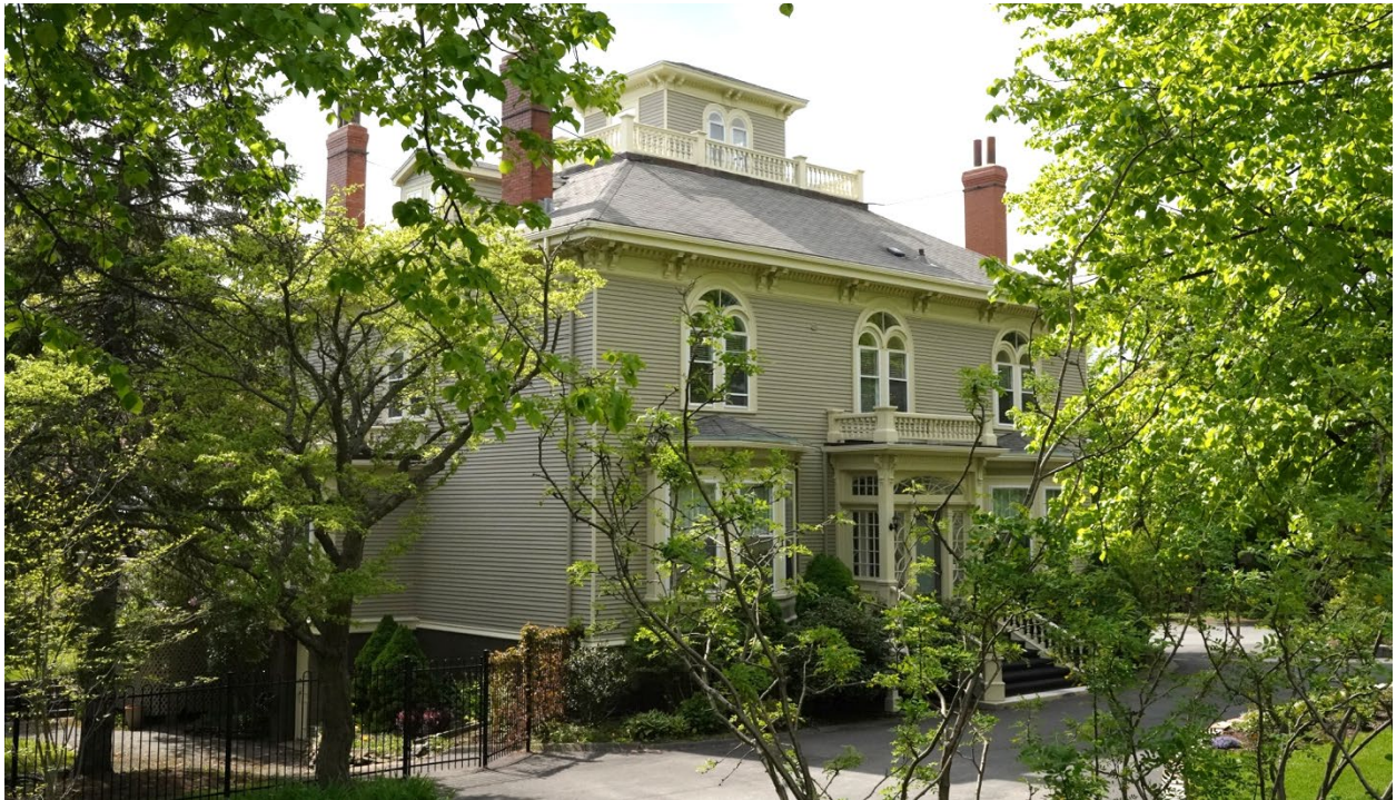
Figure 17: Southeast elevation (May 30, 2022)
