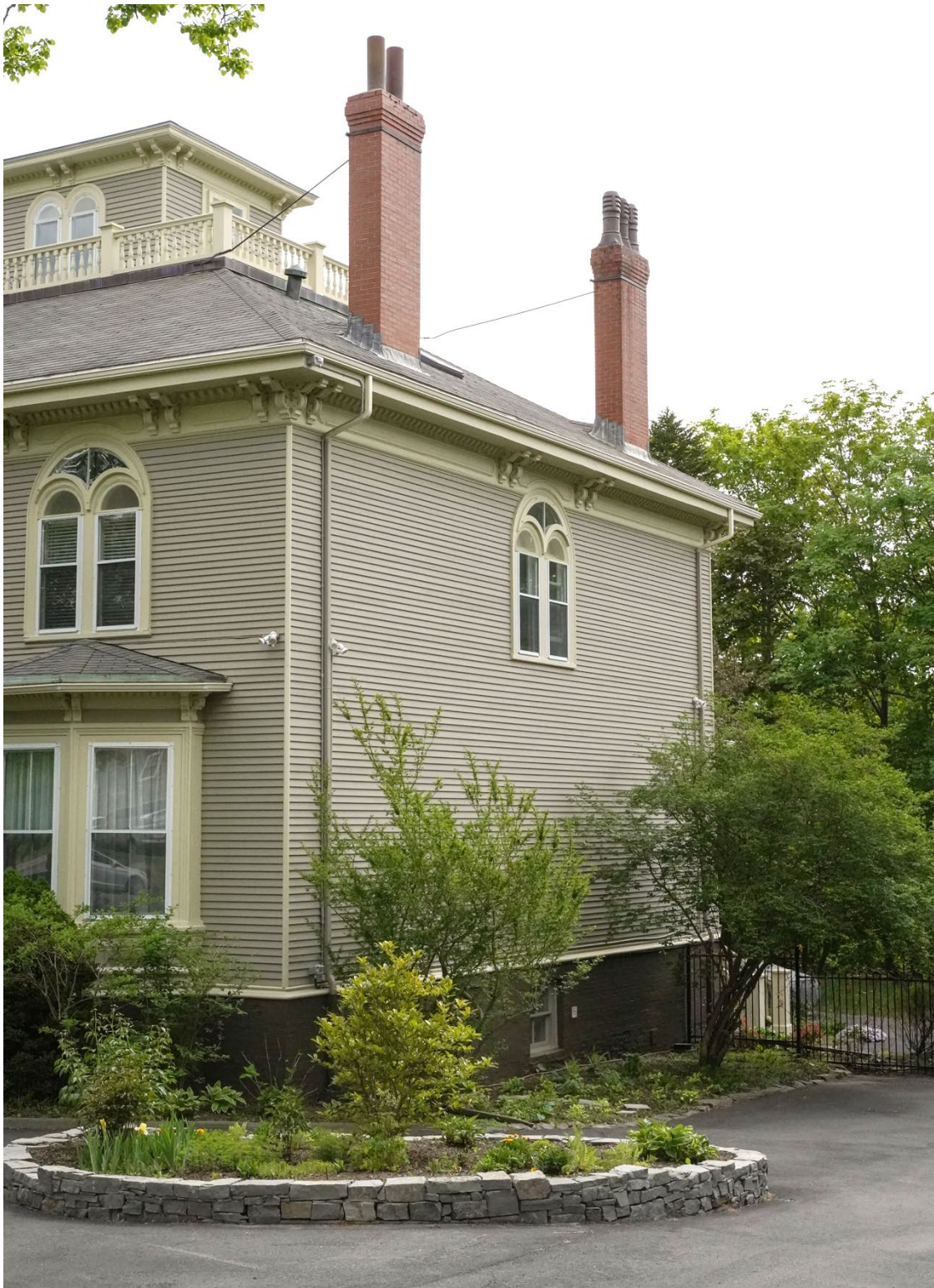
Figure 18: Northern elevation as viewed from the northeast (May 30, 2022)
