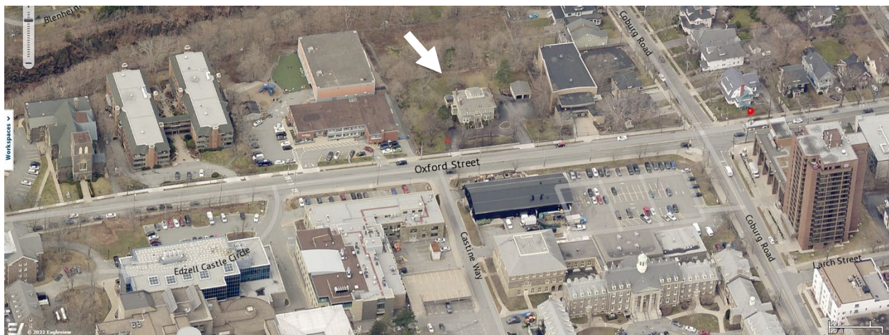
Figure 24: Aerial pictometry of the immediate surroundings looking East [1460 Oxford Street highlighted by a white arrow] (April 12, 2022).
