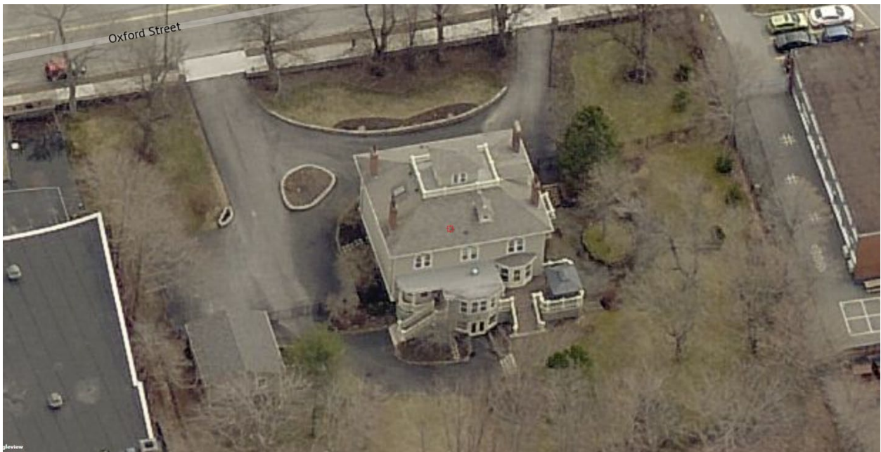
Figure 22: Aerial pictometry of the rear elevation of 1460 Oxford Street (April 12, 2022)
