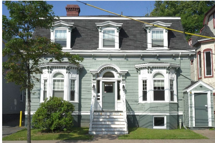
Figure 1: Western elevation of 1322 Robie Street in July 2022
