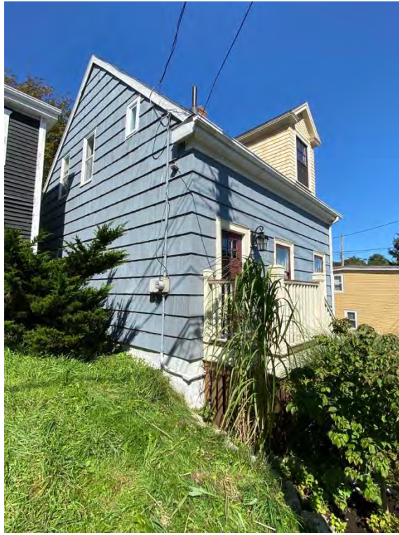
Figure 20: West and south elevations of 65 Tulip Street (05 October 2021)
