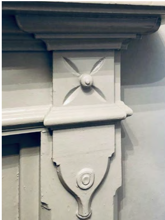
Figure 8: Decorative trim on the upstairs fireplace mantle
