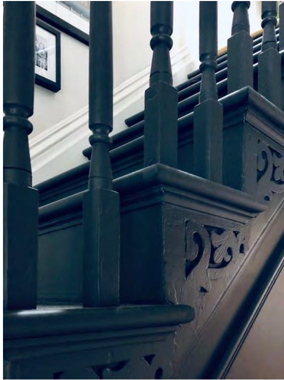
Figure 9: Decorative trim on the stairs and spun spindles
