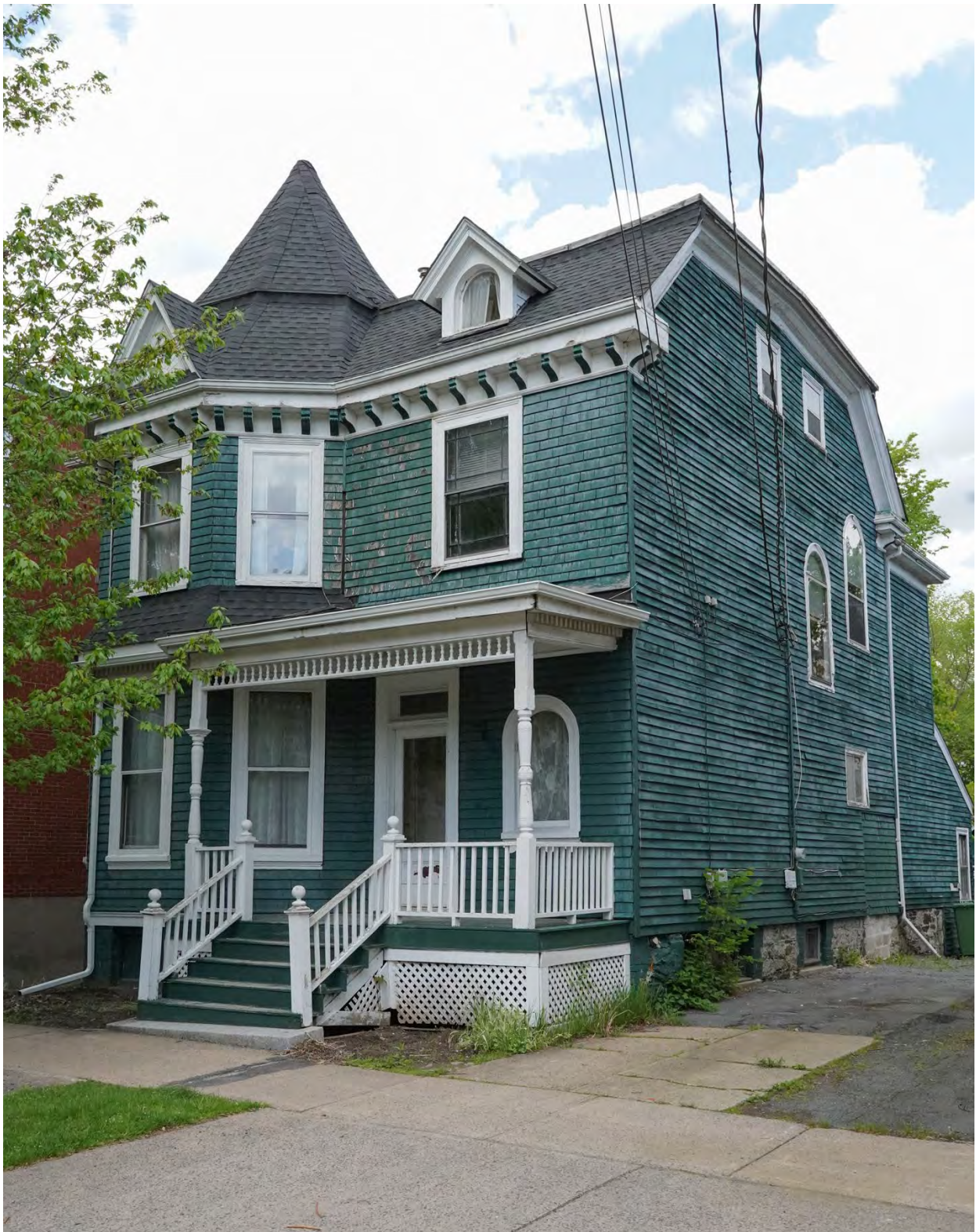
Figure 18: Western elevation as viewed from the southwest (May 30, 2022).
