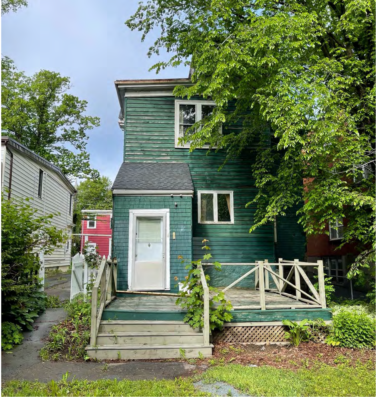
Figure 21: Eastern elevation (June 10, 2022).
