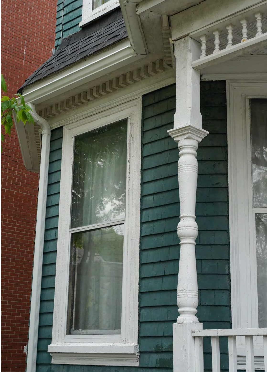
Figure 24: Detail of bay window, turned veranda post with capital, dentils, and spandrels (May 30, 2022).
