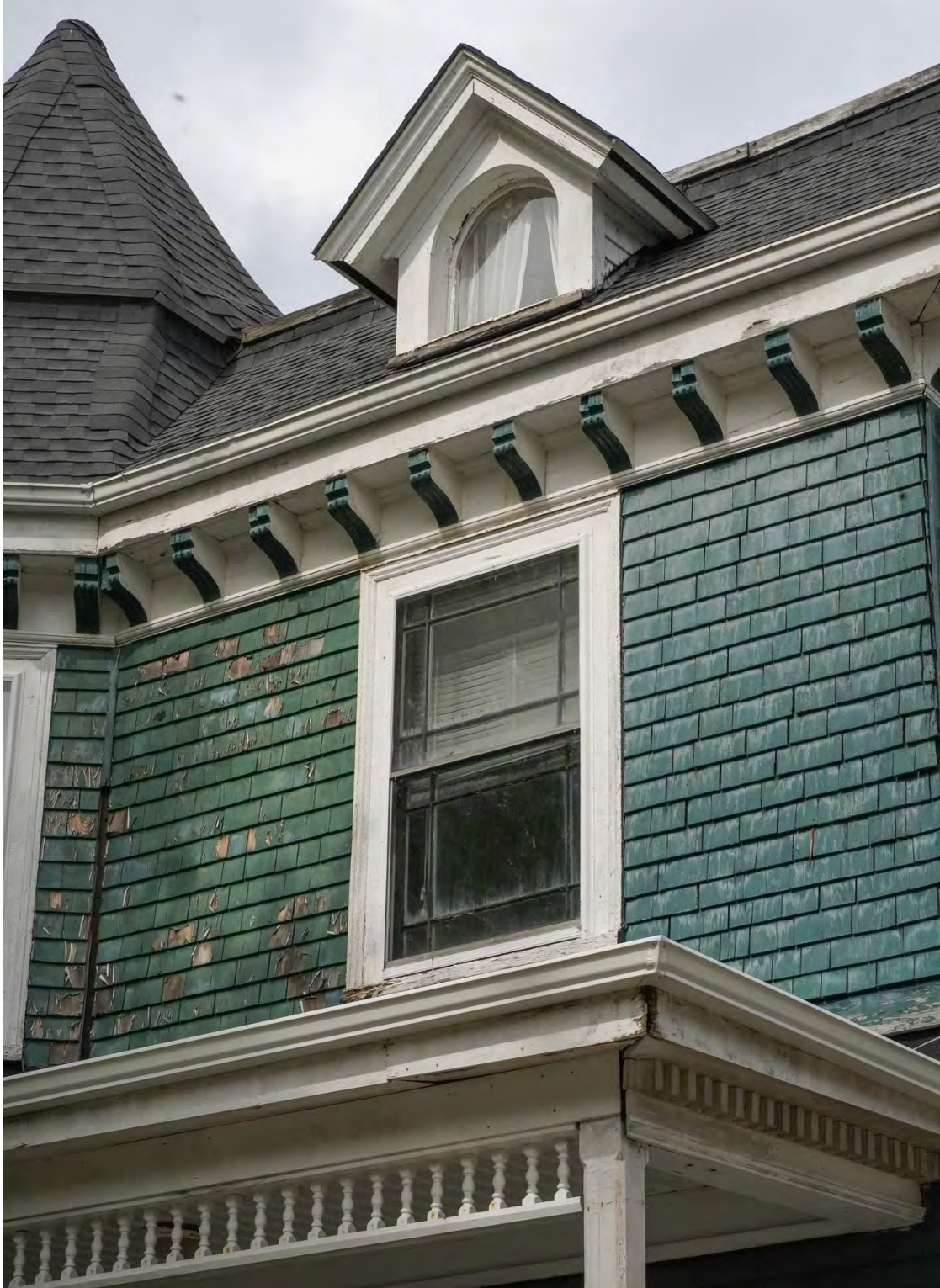
Figure 23: Detail of prairie-style muntins, dormer, bracketed cornice, and spandrels (May 30, 2022).
