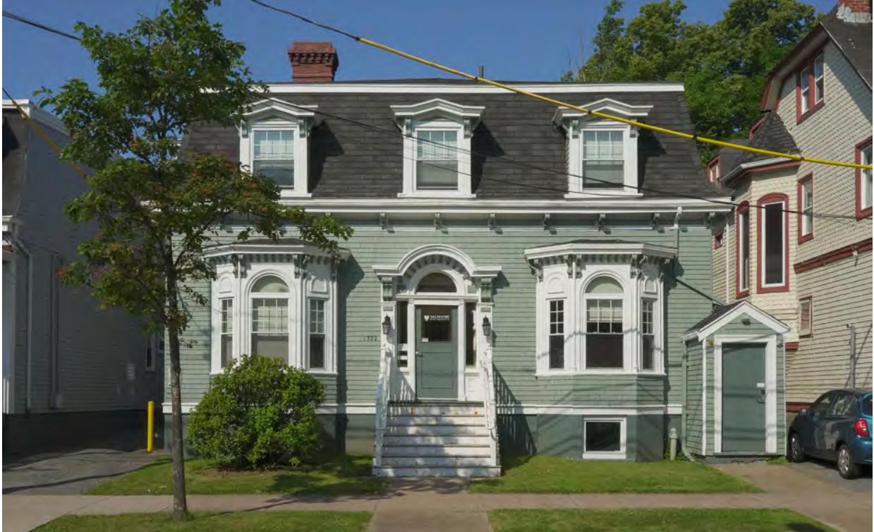
Figure 15: Eastern Elevation (July 21, 2022)
