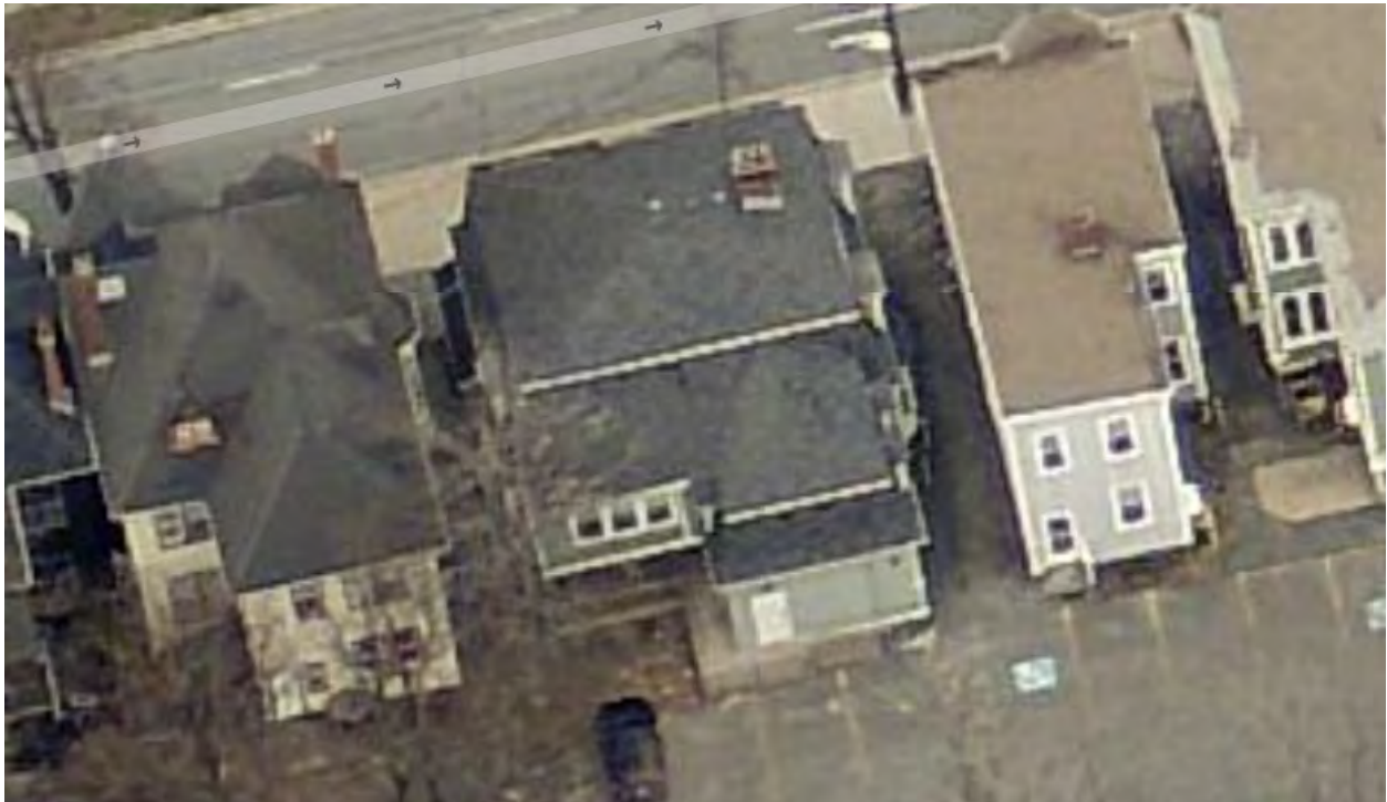
Figure 16: Western Elevation as seen in aerial pictometry (April 26, 2020)
