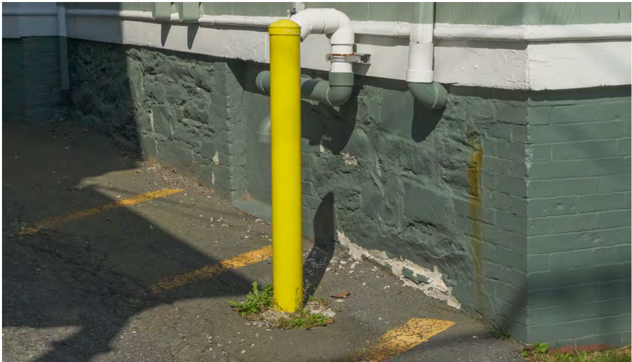
Figure 20: Detail of the brick and coursed rubble foundations (July 21, 2022)
