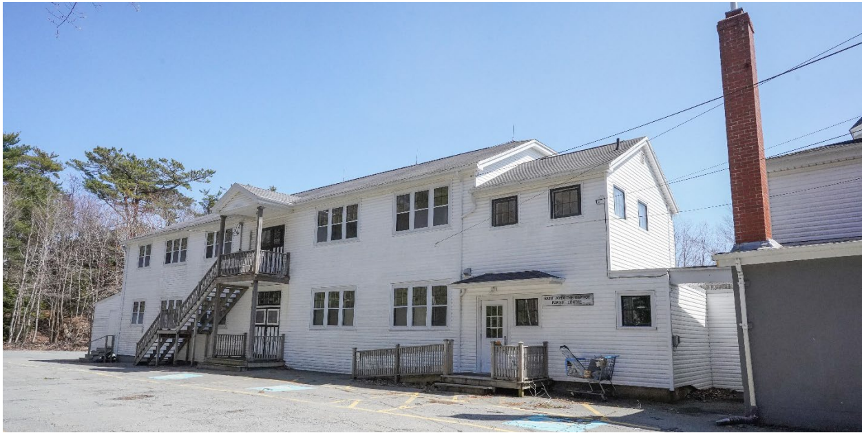
Figure 24: Sister Pius Memorial School at the rear of the church (May 3, 2022)
