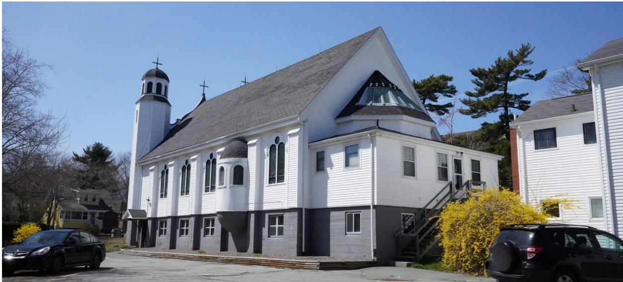
Figure 22: Southeast elevation showing the apse skylight and oriel window (May 3, 2022)
