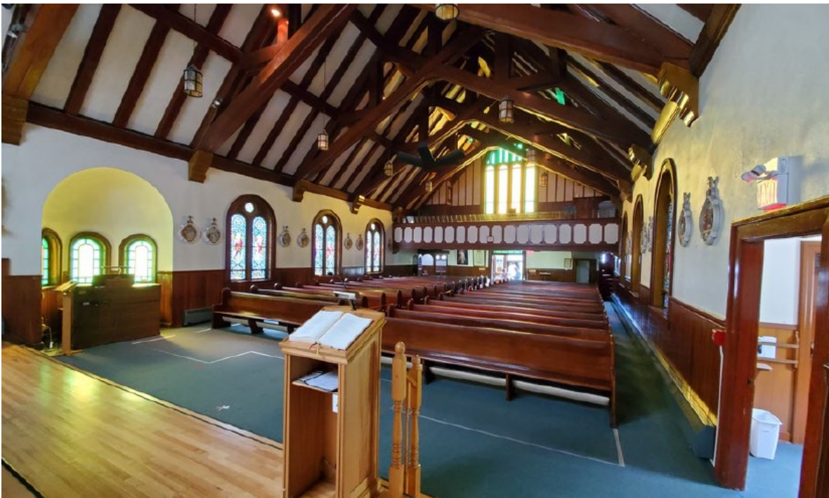
Figure 26: Interior of the church looking west towards the entrance [February 2022] (FBM Consulting, 2022)
