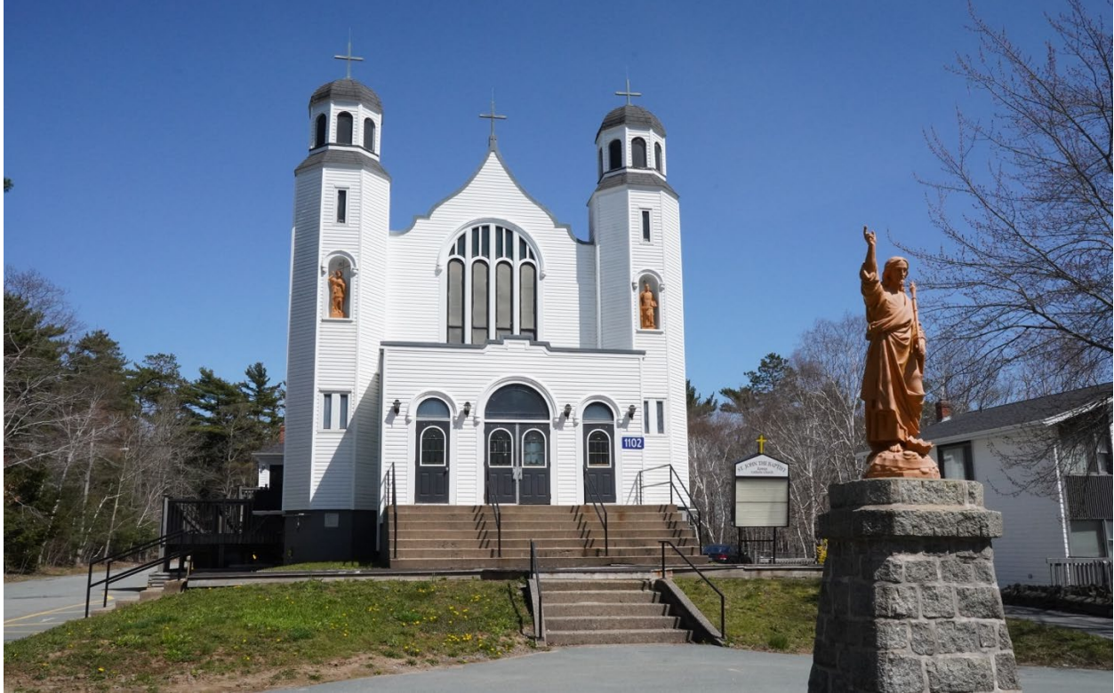
Figure 19: Western elevation (May 3, 2022)
