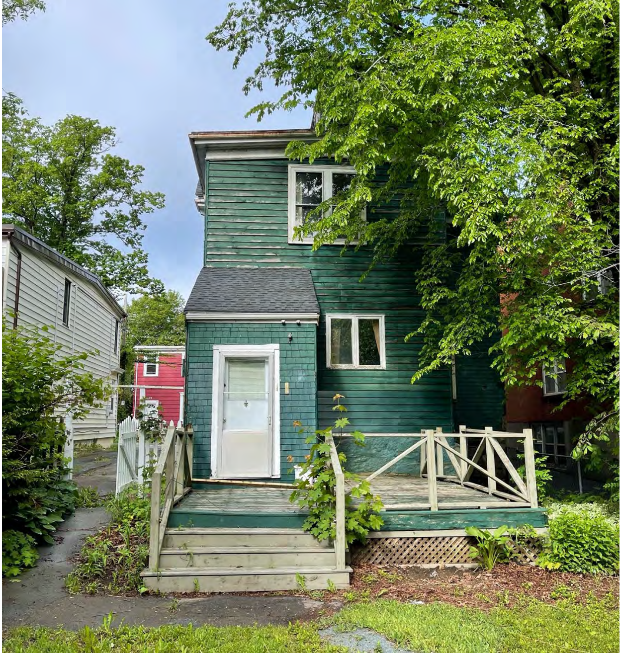
Figure 21: Eastern elevation (June 10, 2022).
