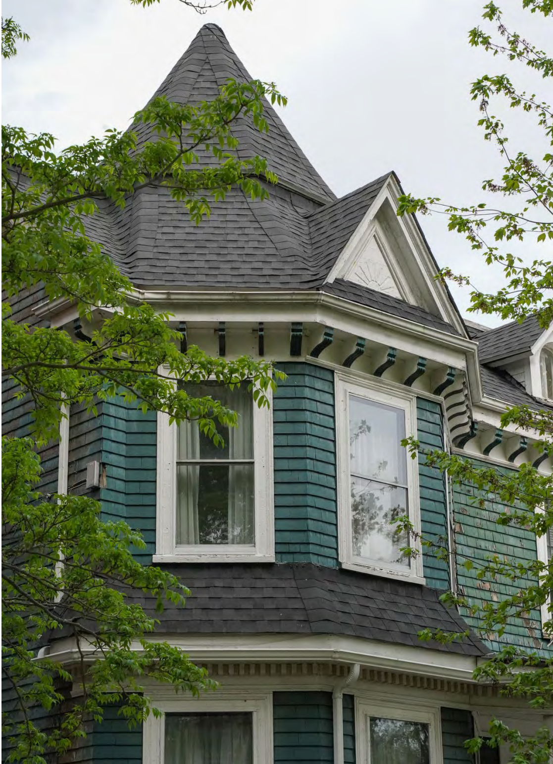
Figure 22: Detail of the two-story bay window, dentils, bracketed cornice, octagonal roof turret, and sunburst gable (May 30, 2022).
