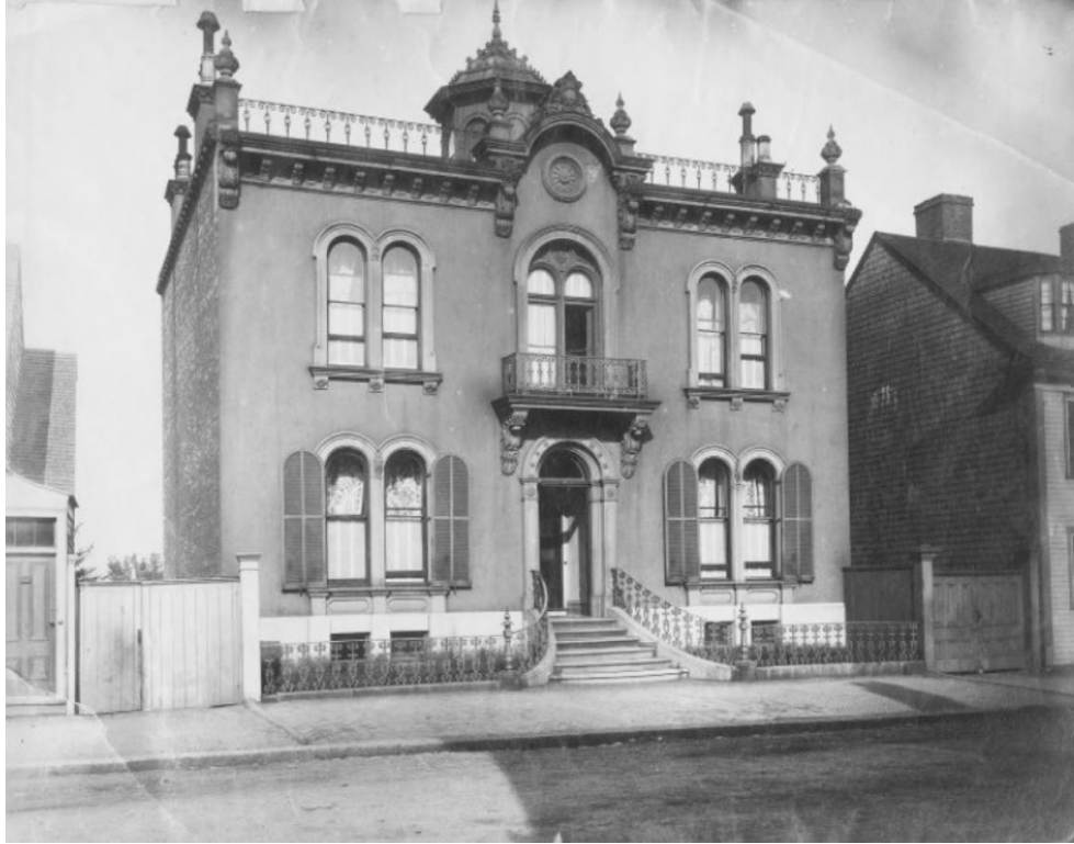
Figure 20: West elevation of 2287 Brunswick Street c. 1880 showing original roofline (Notman Studio, 1880)
