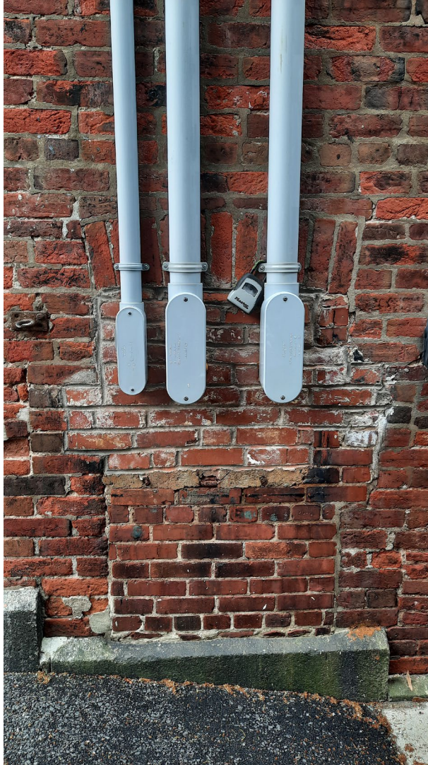
Figure 24: Blinded window on the south elevation (July 17, 2021)
