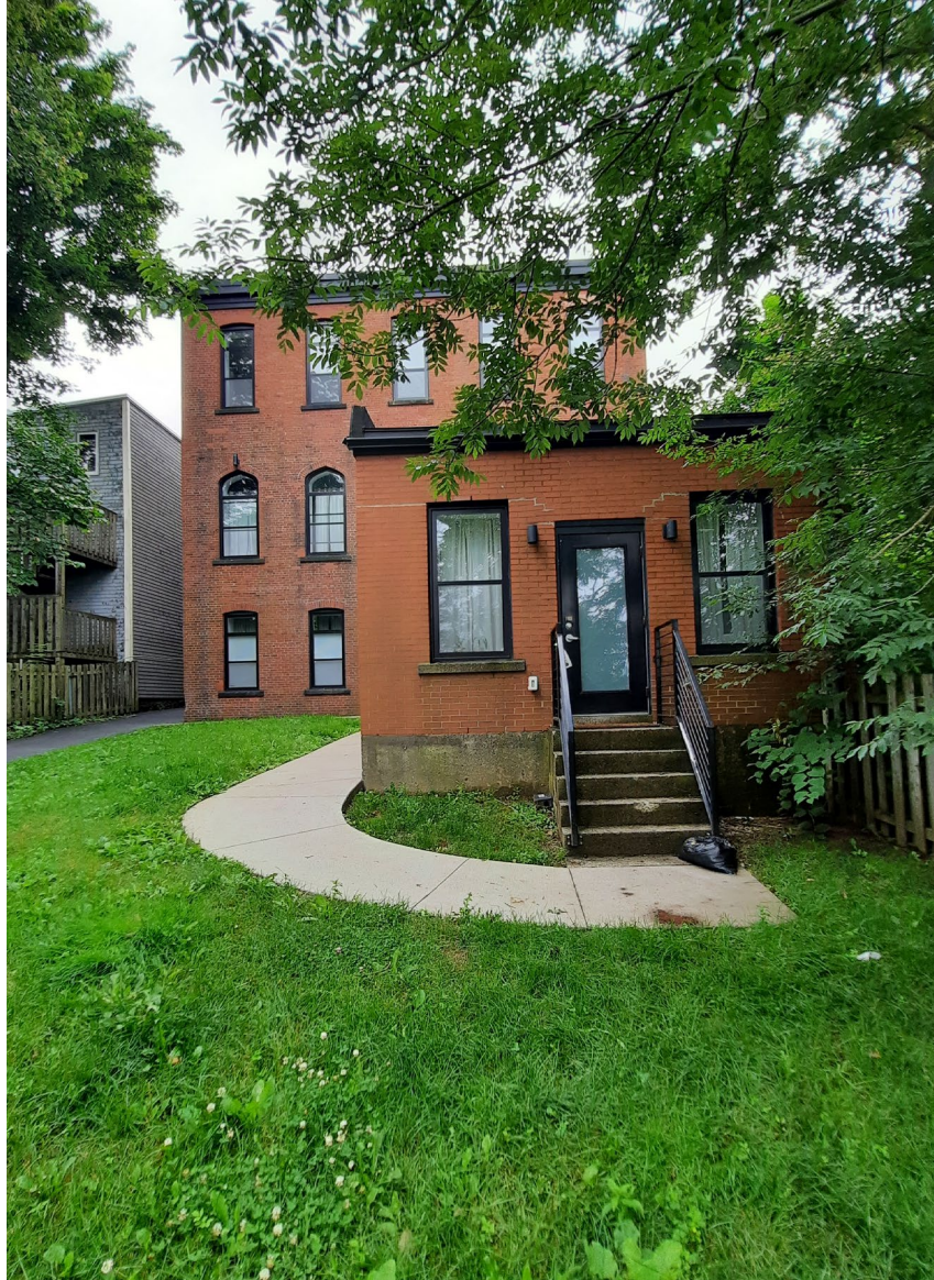
Figure 15: East elevation (July 17, 2021)
