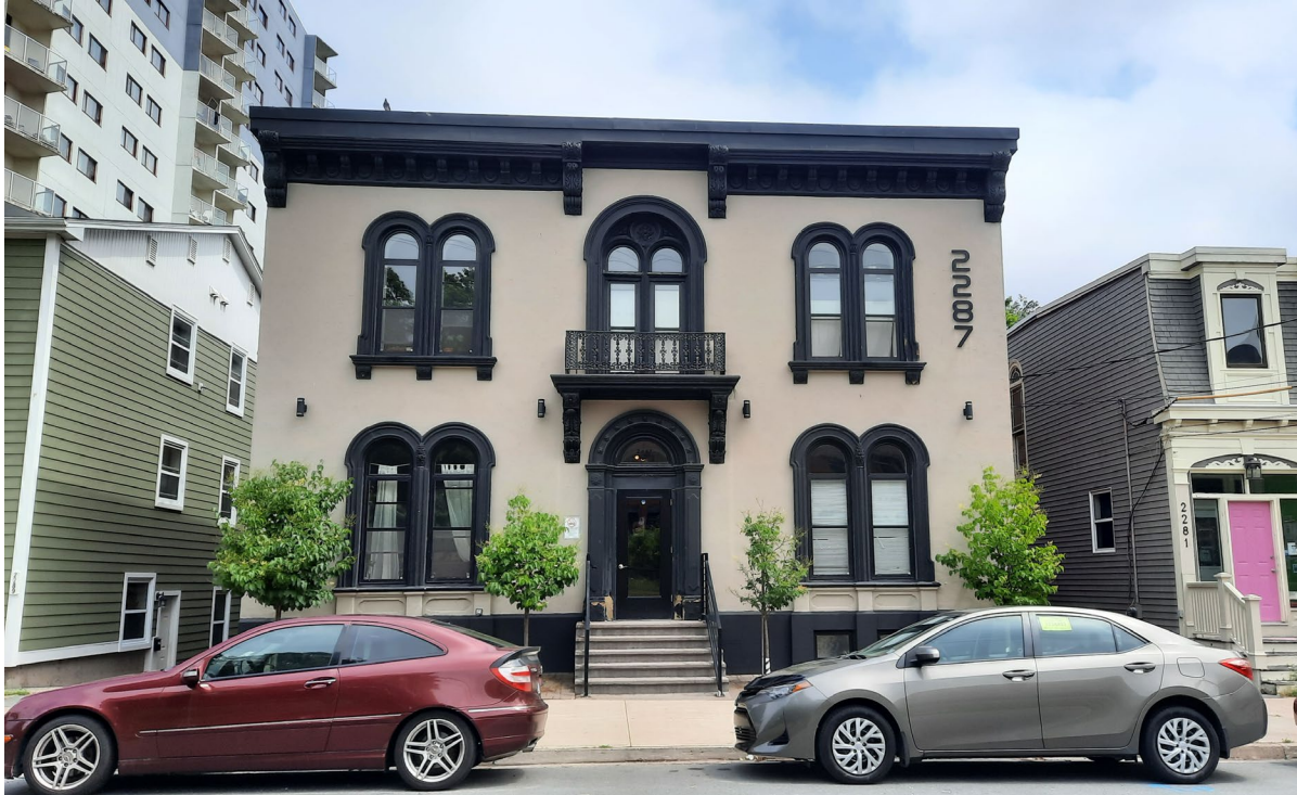
Figure 11: West elevation of 2287 Brunswick Street (July 17, 2021)
