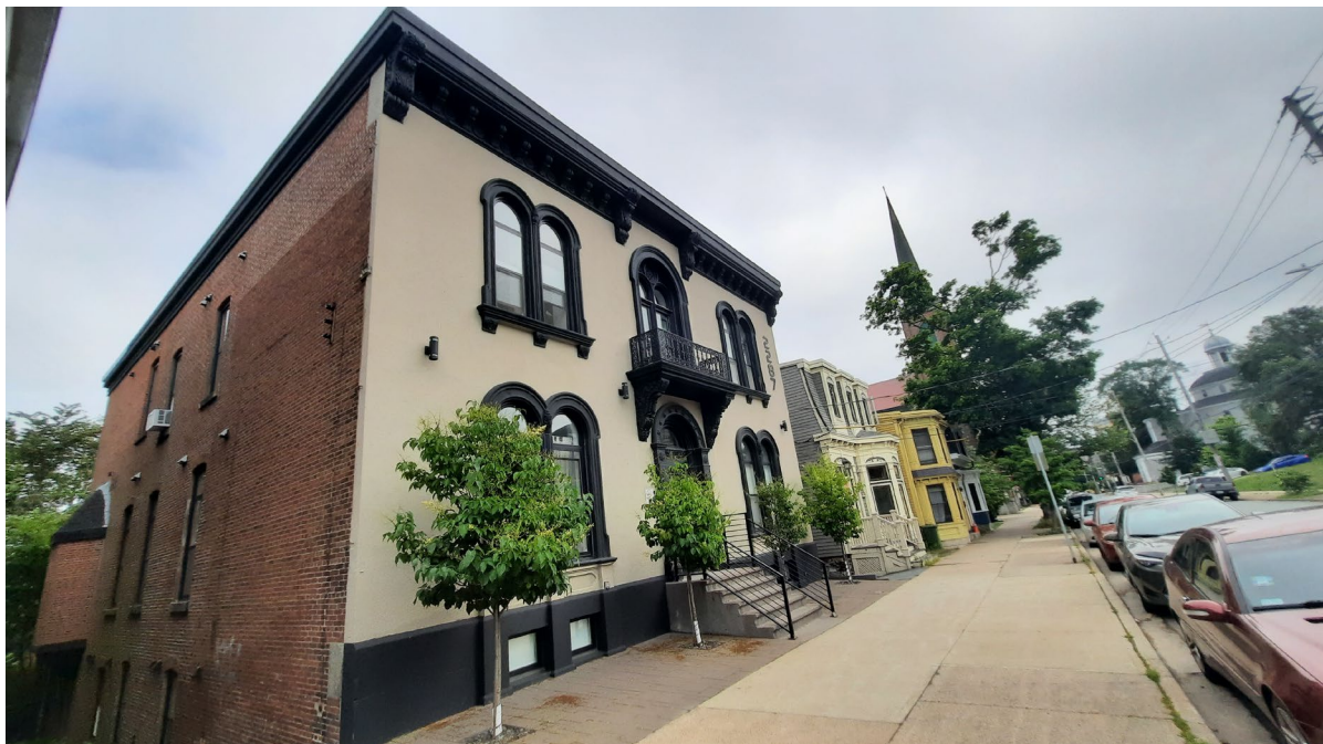
Figure 12: West and north elevations of 2287 Brunswick Street (July 17, 2021)
