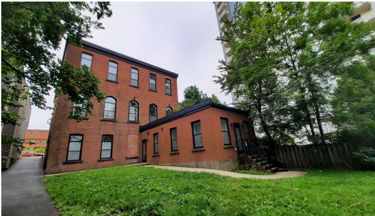
Figure 14: East and south elevations of 2287 Brunswick Street (July 17, 2021)
