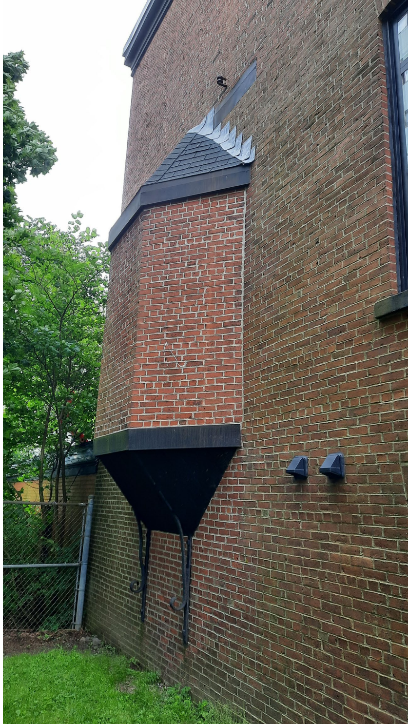
Figure 17: Oriel window on the north elevation (July 17, 2021)
