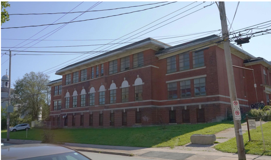
Figure 28: St. Patrick's Boys School, located opposite the church and rectory [2326 Brunswick Street] (September 20, 2021)
