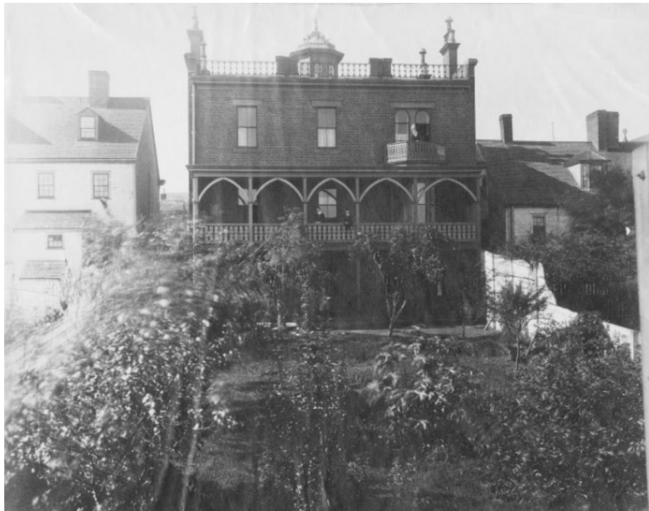
Figure 21: East elevation of 2287 Brunswick Street, undated [est. 1880] showing original roofline and rear balcony (Notman Studio, n.d.)
