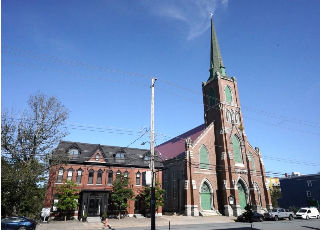
Figure 27: St. Patrick's Catholic Church and Rectory [2263 & 2267 Brunswick Street] (September 20, 2021)
