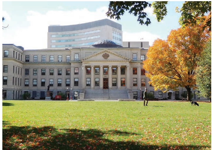
Pictured above: Tabaret Hall, protected under the Sandy Hill West HCD
