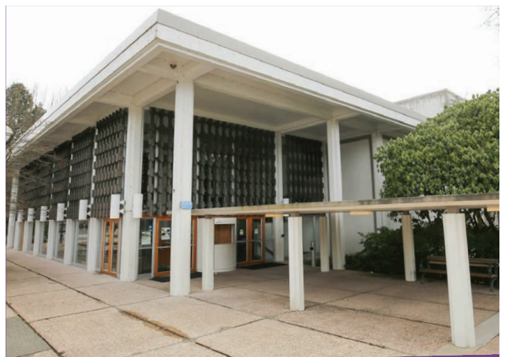
Pictured above: Frederick Wood Theatre (unprotected)
