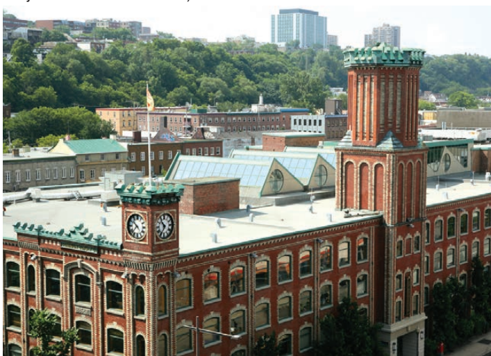
Pictured above: Édifice la Fabrique (national historic site, under the jurisdiction of the CUQC)
