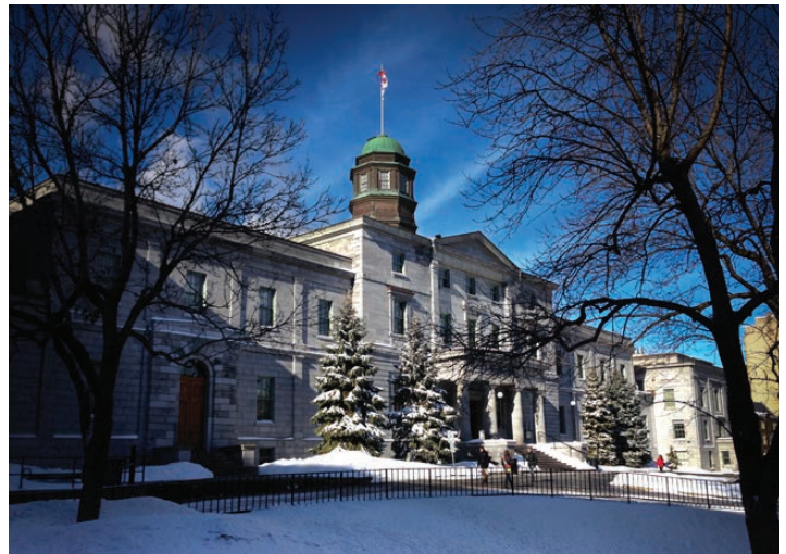
Pictured above: Dawson Hall, protected by HCD and the Mount Royal provincial heritage site.
