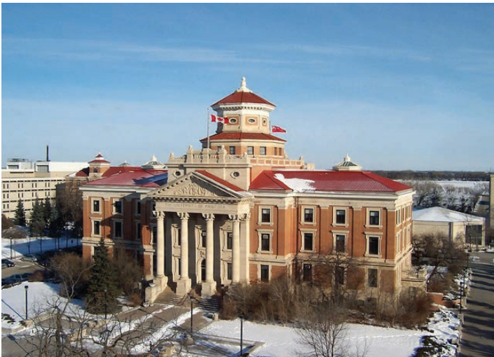
Pictured above: Administration Building (designated)
