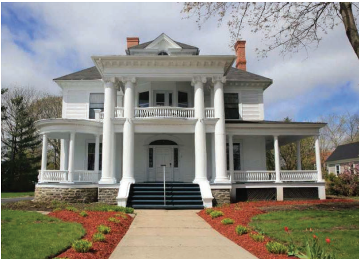
Pictured above: 58 Waterloo Row (former university president's residence) located within the Saint Anne's Point Preservation Area
