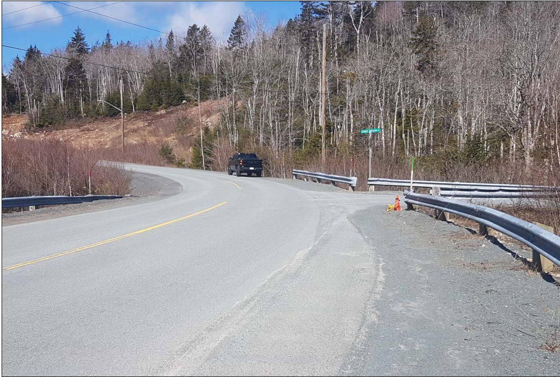
Winslow Drive – Looking North through Earl Retson Drive Intersection
