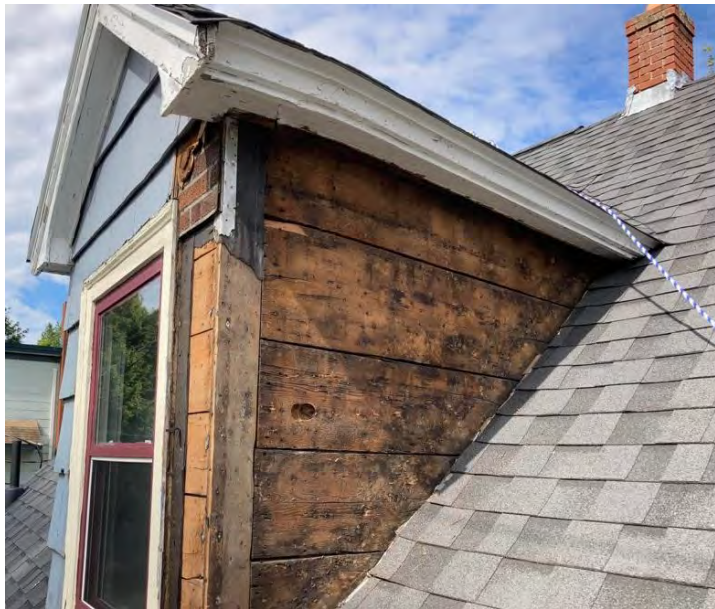
Figure 21: Evidence of Scottish dormer (22 September 2021)
