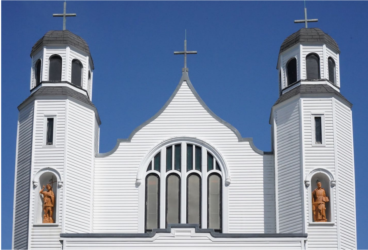
Figure 23: Closeup of Spanish Mission Revival details, including decoratively shaped parapets and Moorish octagonal belltowers (May 3, 2022)
