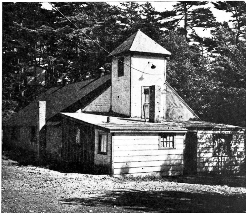
THE OLD CHURCH—NOW FITTED UP AS AN A.R.P. EMERGENCY HOSPITAL
