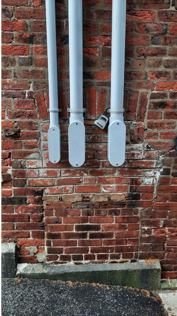
Figure 24: Blinded window on the south elevation (July 17, 2021)
