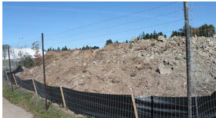
Construction & Silt fence (Figure F3)
