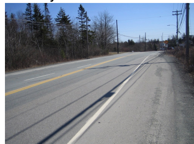
Photo 4 - Looking east on Sackville Drive towards the Margeson Drive roundabout from proposed driveway for ground level parking area.
