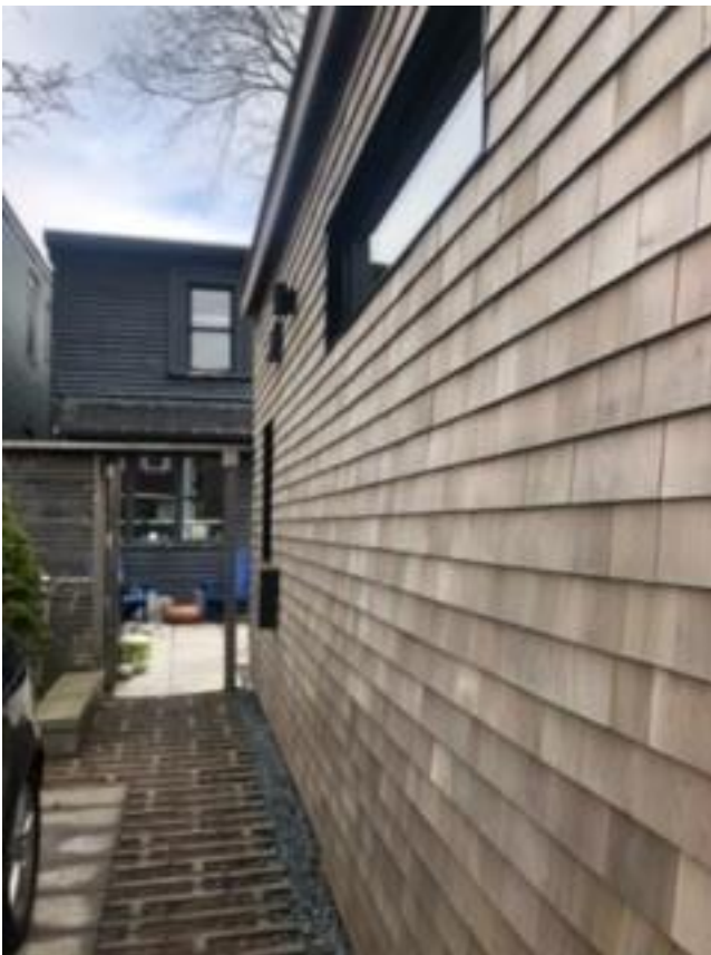
2376 Moran Street showing addition + outbuilding
