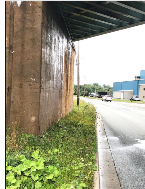
Pinch Point - CN Rail Crossing Near Belmont Avenue
