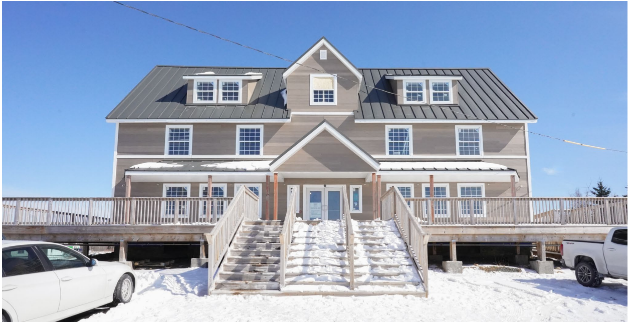
Figure 10: Western elevation of the Old Home (March 1, 2022)
