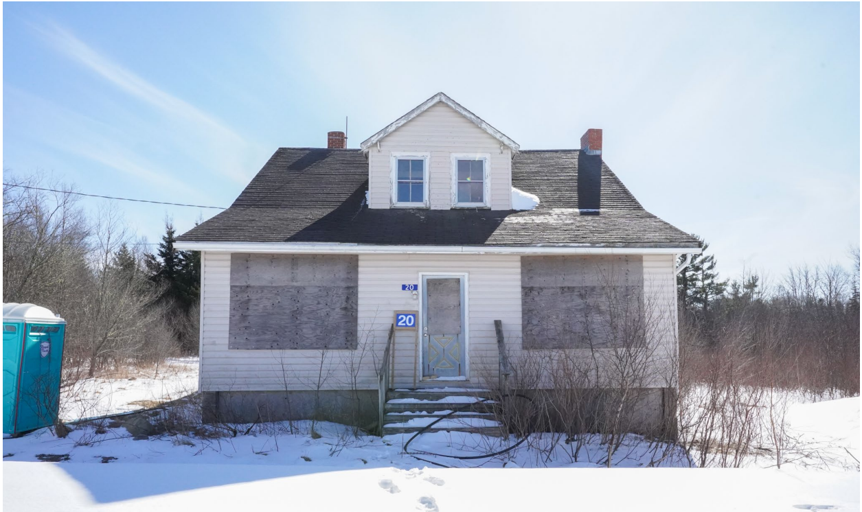
Figure 14: Outbuilding at 20 Wilfred Jackson Way (March 1, 2022)
