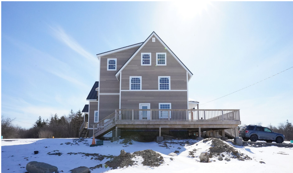
Figure 13: Northern elevation of the Old Home (March 1, 2022)
