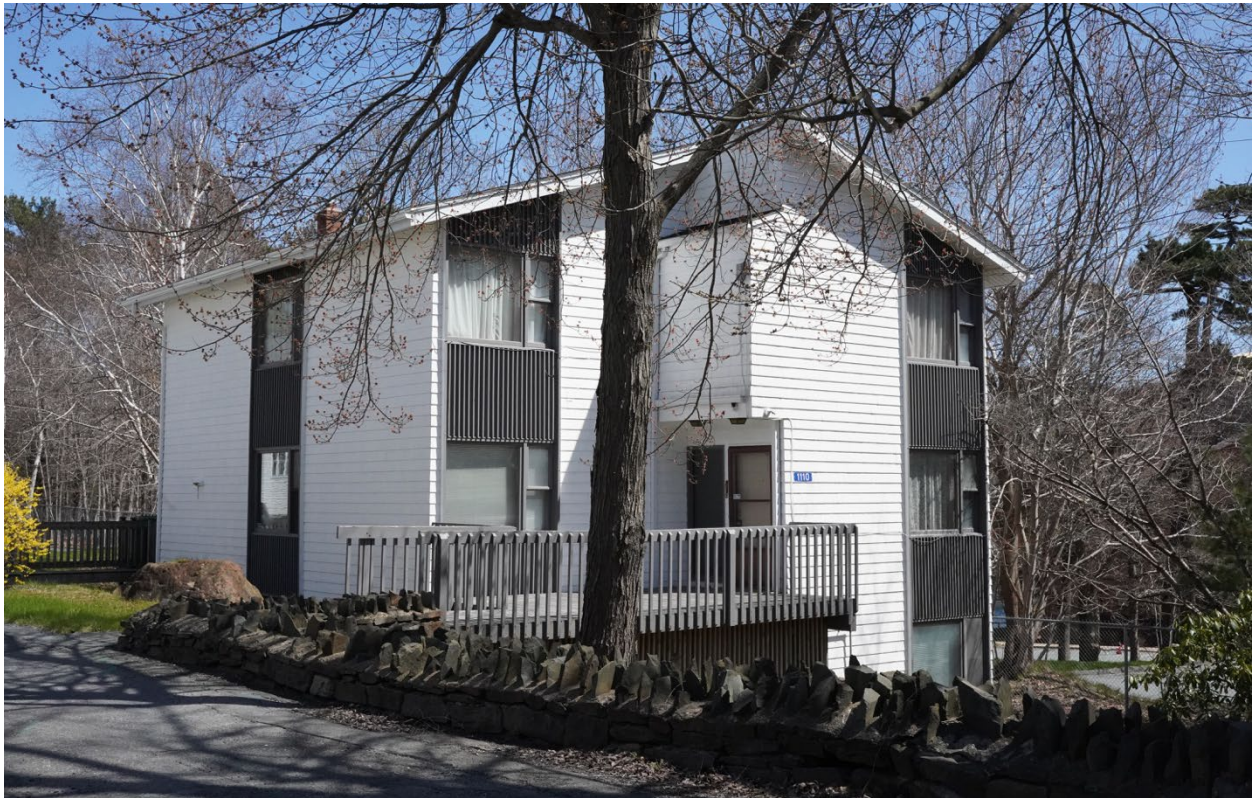
Figure 34: The new rectory located to the south of the church (May 3, 2022)
