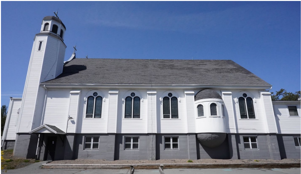
Figure 20: Southern elevation (May 3, 2022)
