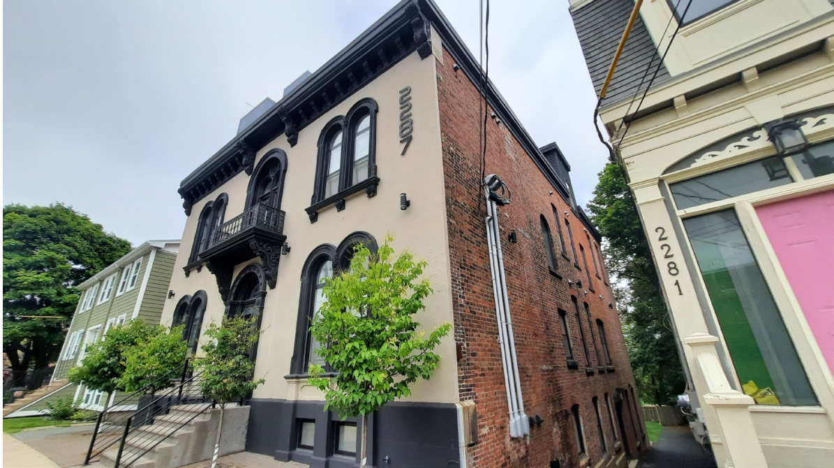
Figure 13: West and south elevations of 2287 Brunswick Street (July 17, 2021)
