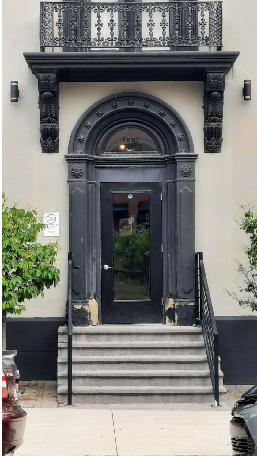
Figure 16: Main entrance on the west elevation (July 17, 2021)
