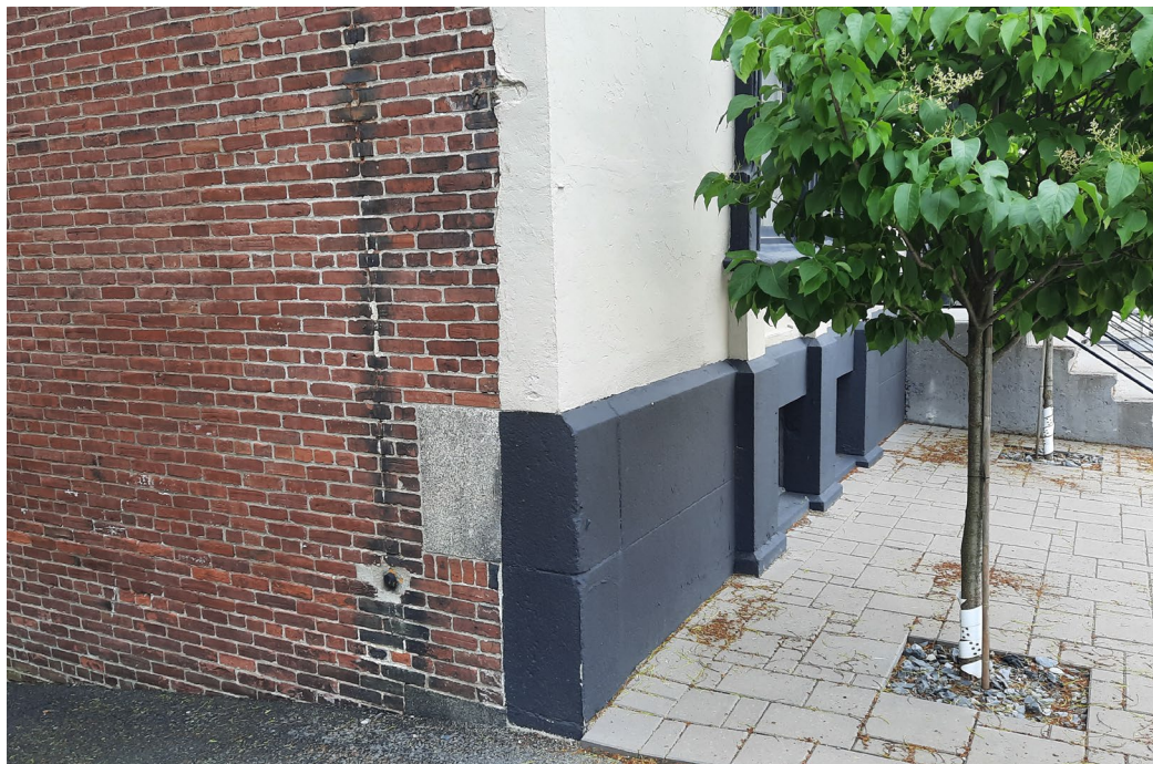
Figure 23: Painted black granite foundation with evidence of original granite to the left (July 17, 2021)
