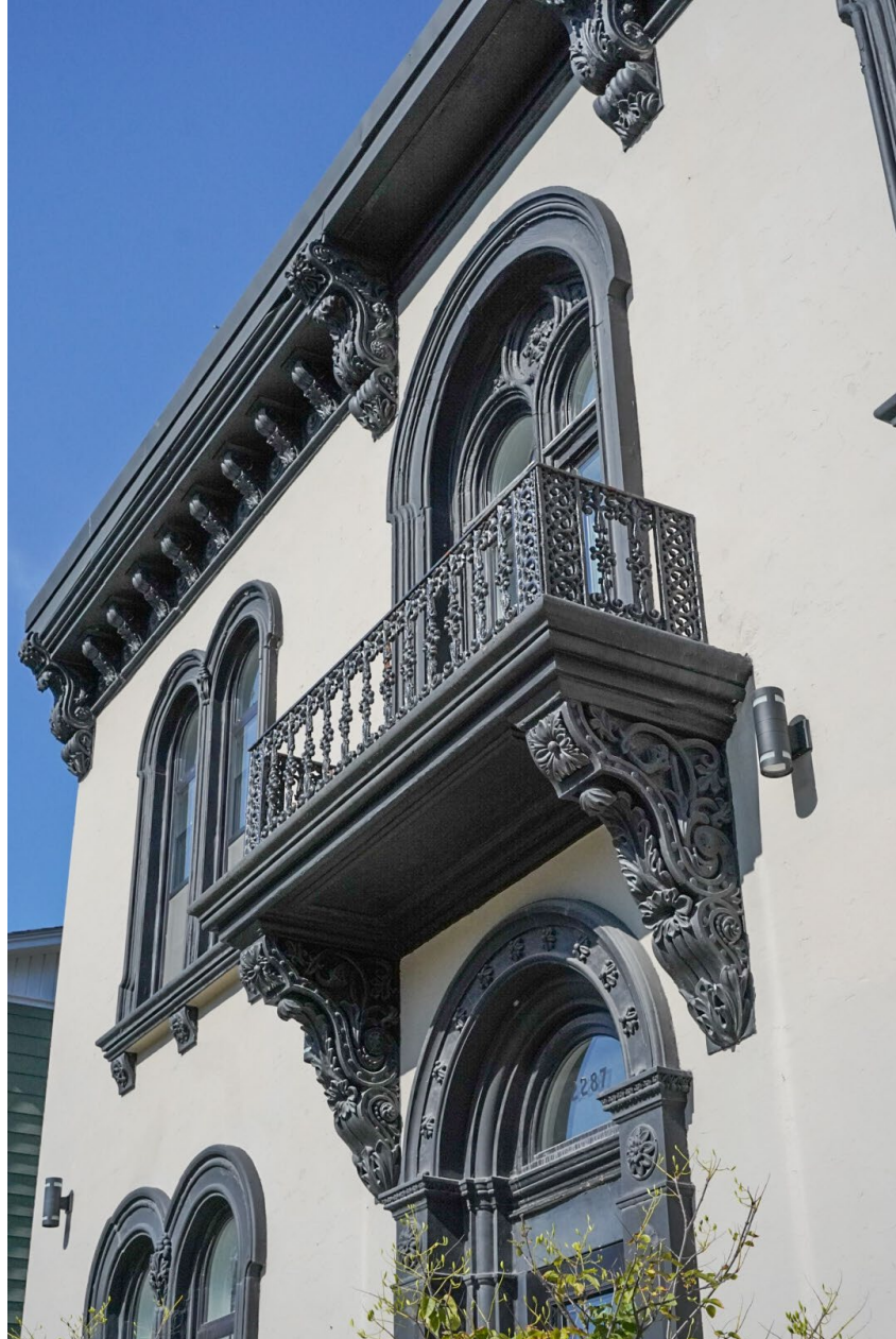
Figure 18: Detail view of balcony and cornice (September 20, 2021)
