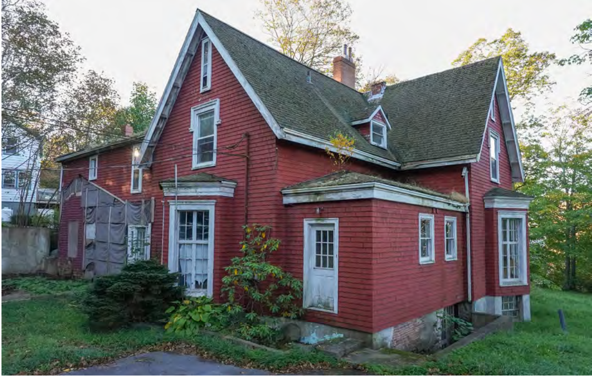
Figure 11: Northeastern elevation of 144 Pleasant Street (October 19, 2021)
