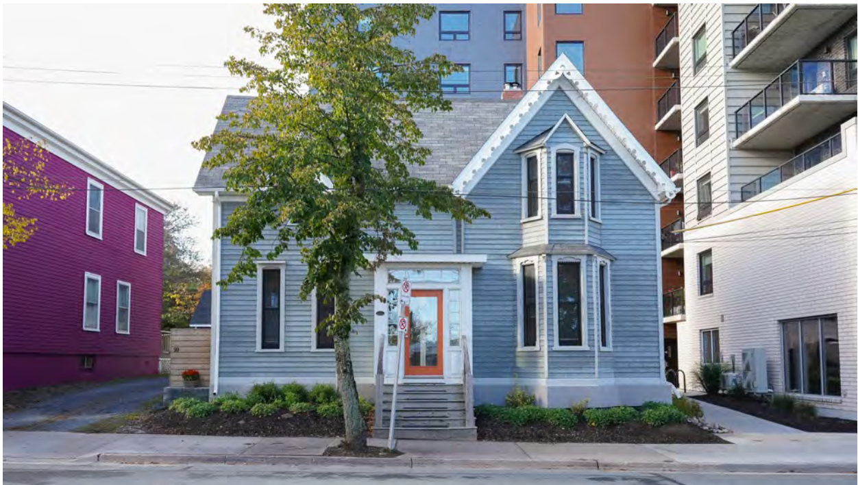
Figure 33: Henry Elliot House [99 Ochterloney Street] (November 1, 2021)
