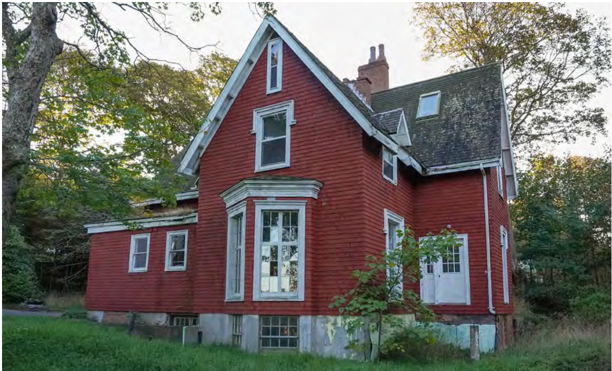
Figure 12: Northwestern elevation of 144 Pleasant Street (October 19, 2021)
