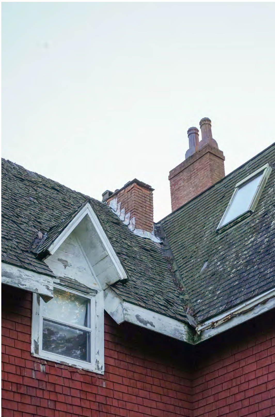
Figure 17: Detail view of western-facing dormer and central chimneys, 144 Pleasant Street (October 19, 2021)
