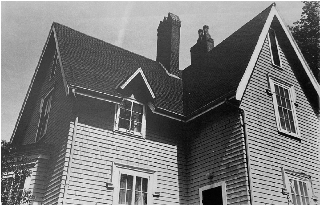
Figure 23: Detail view of west-facing dormer and central chimneys of 144 Pleasant Street est. 1970s-1980s ( Untitled Series of Photographs of 144 Pleasant Street, n.d. )
