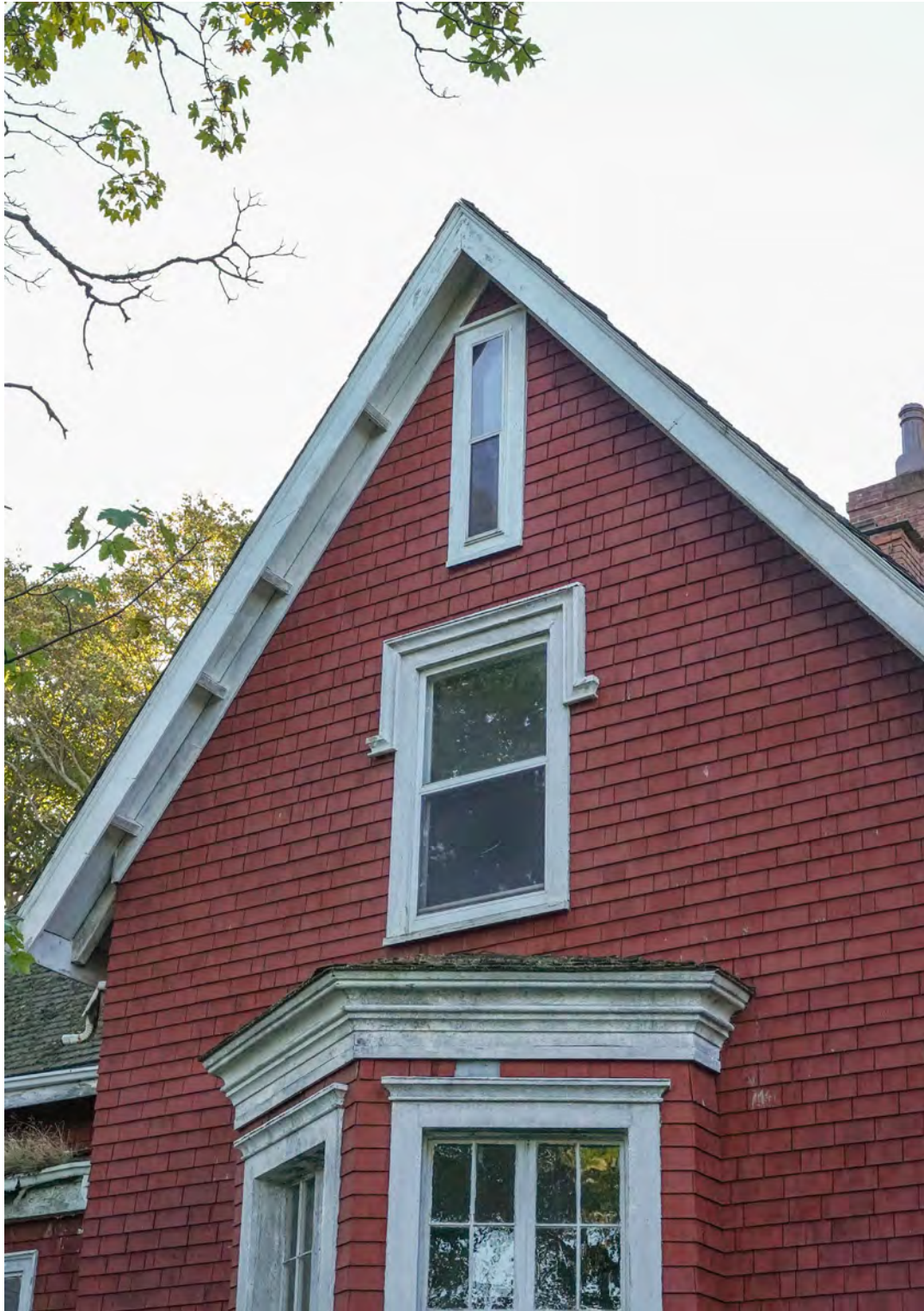
Figure 16: Detail view of northern gable, second-storey window and attic window, 144 Pleasant Street (October 19, 2021)
