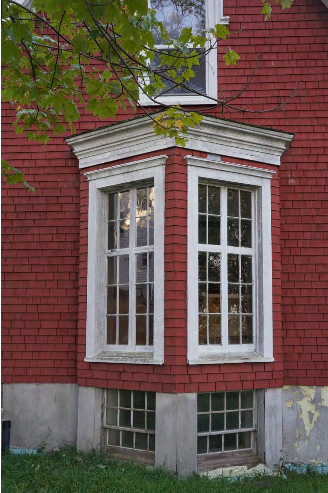
Figure 15: Detail of northern bay window, 144 Pleasant Street (October 19, 2021)
