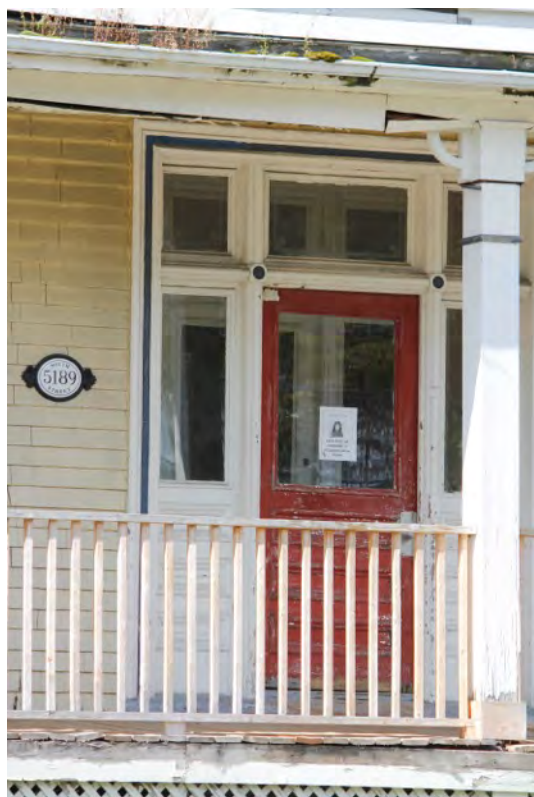
Entry door with sidelights and transom
