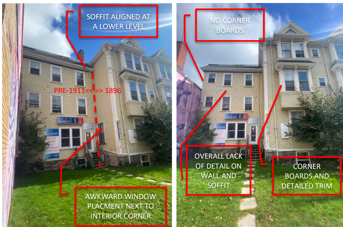
Figure 11a: Components of rear extension that suggest a post-1896 construction date
