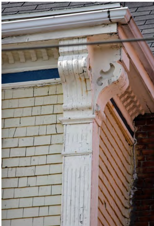
Corner board, top brackets and dentils
