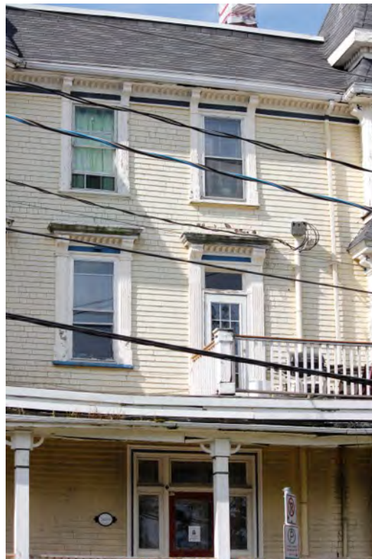
Window and upper door placement, trim and pronounced lintels
