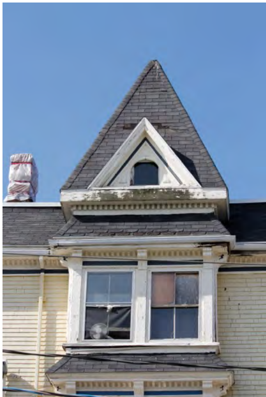
Central roof tower and squared bay
