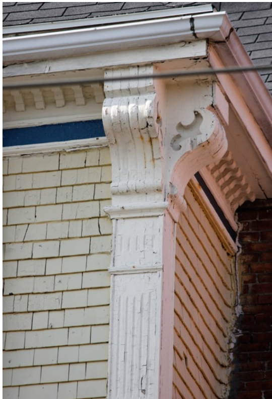
Corner board, top brackets and dentils
