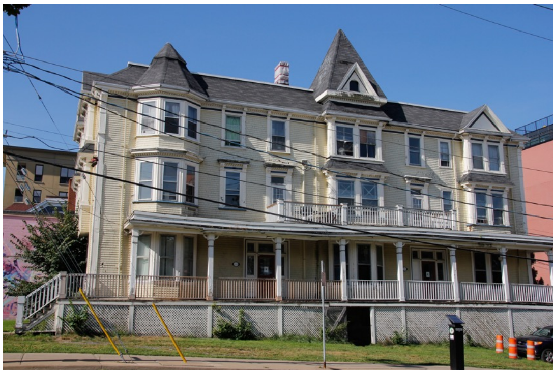
Site overview: south side as seen from South Street.
