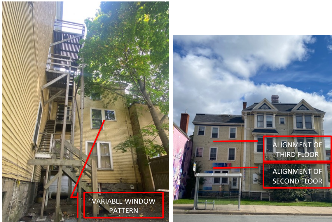
Figure 11b: Components of rear extension that suggest a post-1896 construction date
