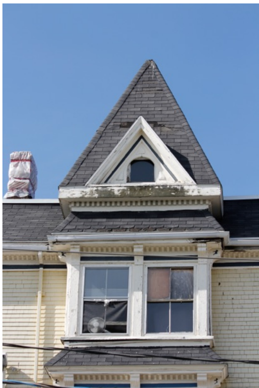
Central roof tower and squared bay
