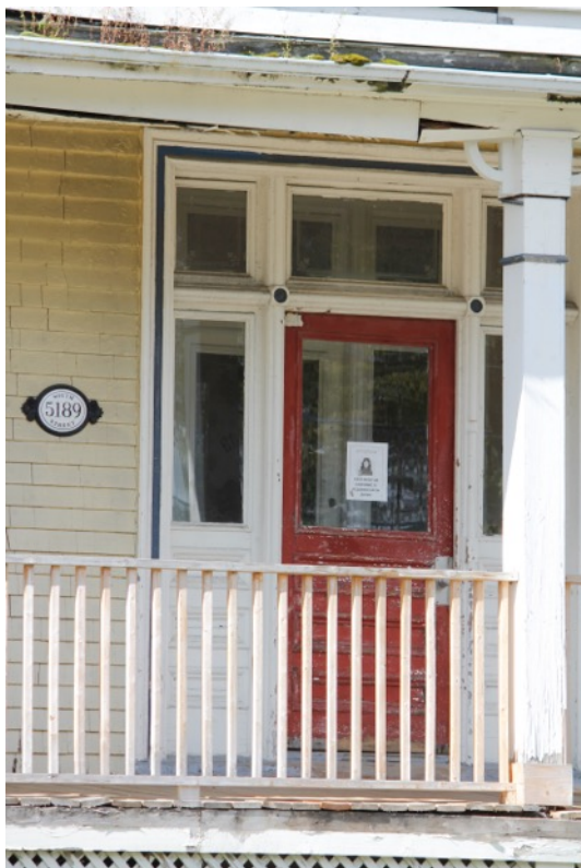
Entry door with sidelights and transom
