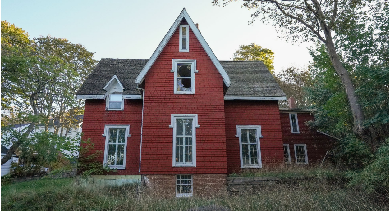
Figure 13: Western elevation of 144 Pleasant Street (October 19, 2021)
