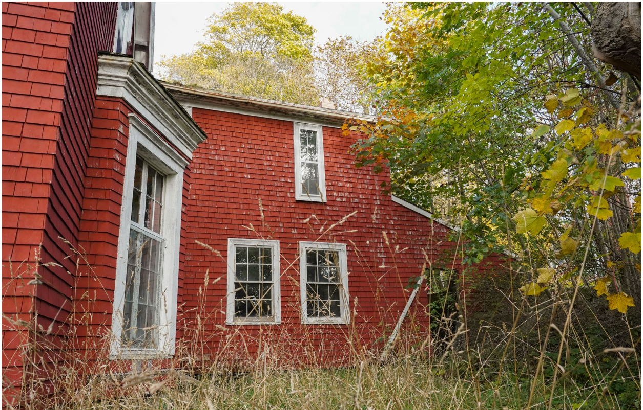
Figure 14: Southern bay window and addition [viewed from the west], 144 Pleasant Street (November 1, 2021)
