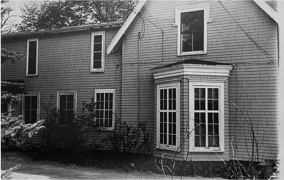
Figure 24: Eastern elevation of 144 Pleasant Street est. 1970s-1980s ( Untitled Series of Photographs of 144 Pleasant Street, n.d. )
