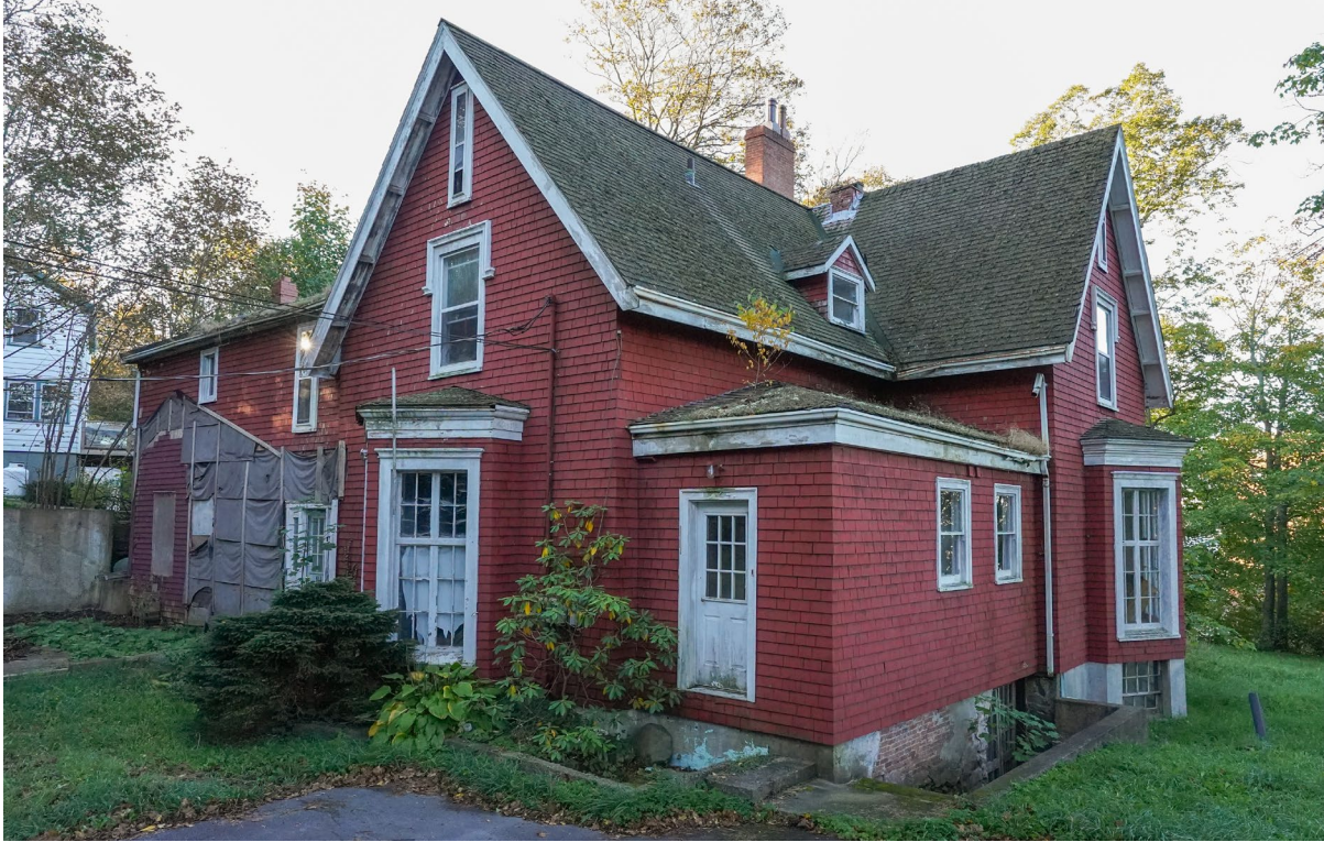
Figure 11: Northeastern elevation of 144 Pleasant Street (October 19, 2021)
