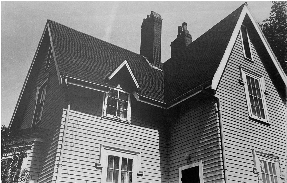
Figure 23: Detail view of west-facing dormer and central chimneys of 144 Pleasant Street est. 1970s-1980s ( Untitled Series of Photographs of 144 Pleasant Street, n.d. )
