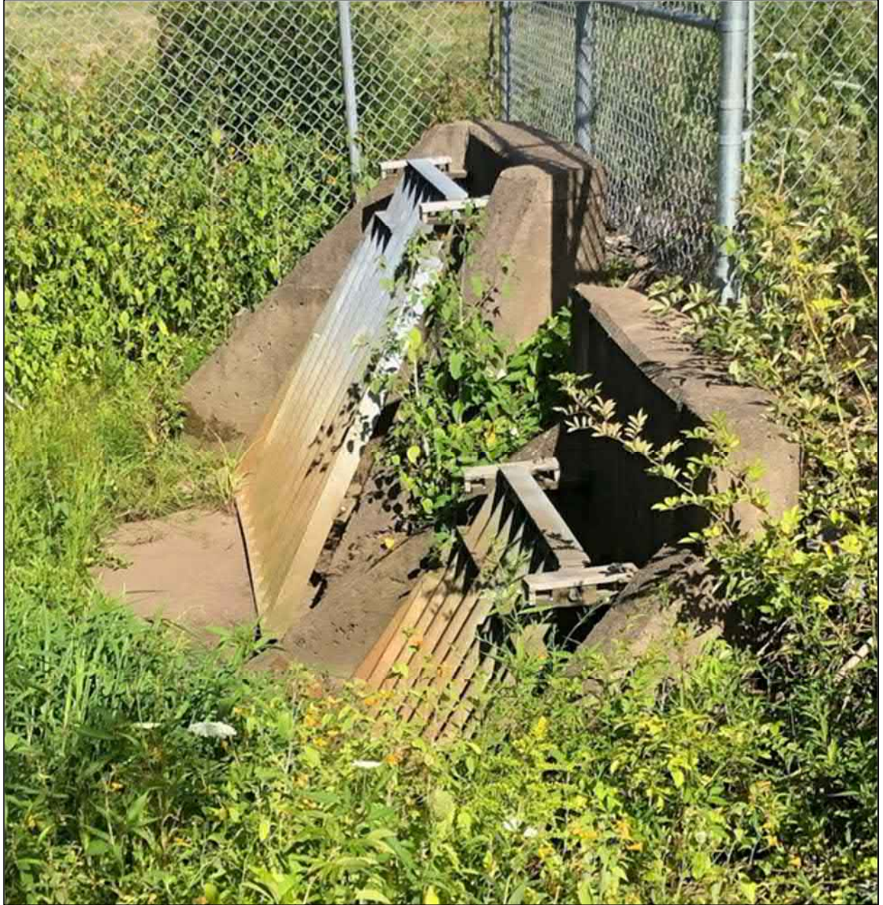
Figure 4-4: Culvert Inlets to Cole Harbour Road
